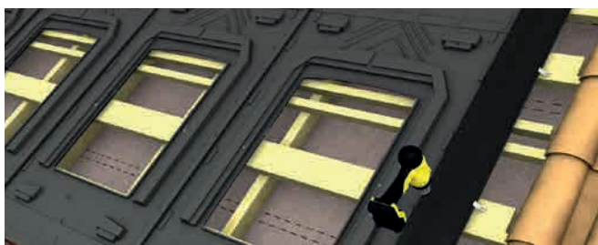
Pre-drilling of GSE frames + flashings + edge wedges
