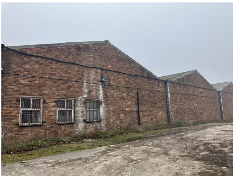
Plate 2 Rear of Existing Warehouse
