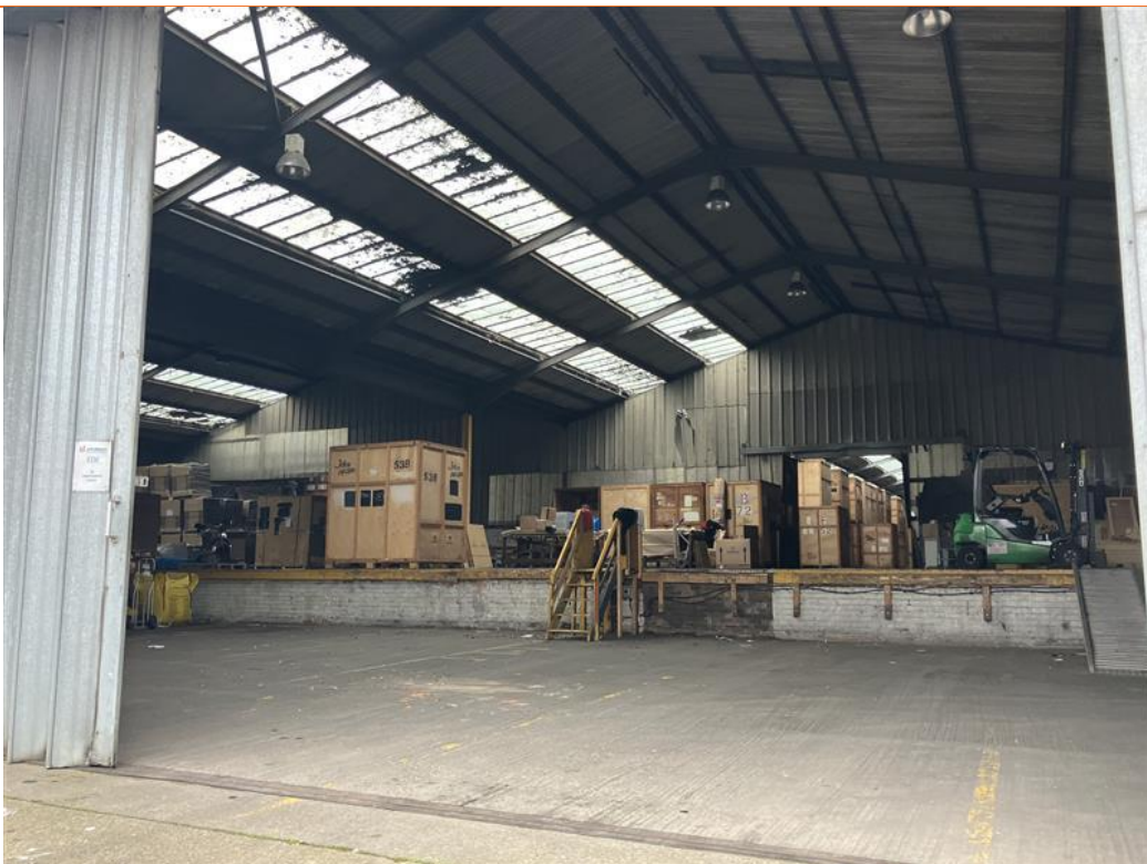
Plate 6 Internal Area of Warehouse
