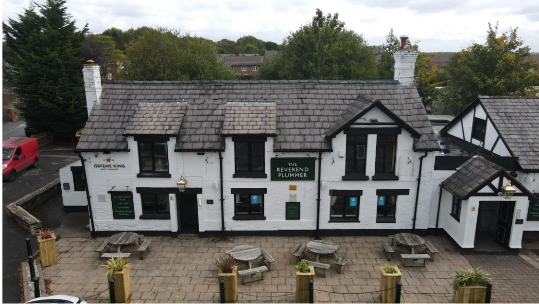
Image 8: Former Reverend Plummer original building c.2020
