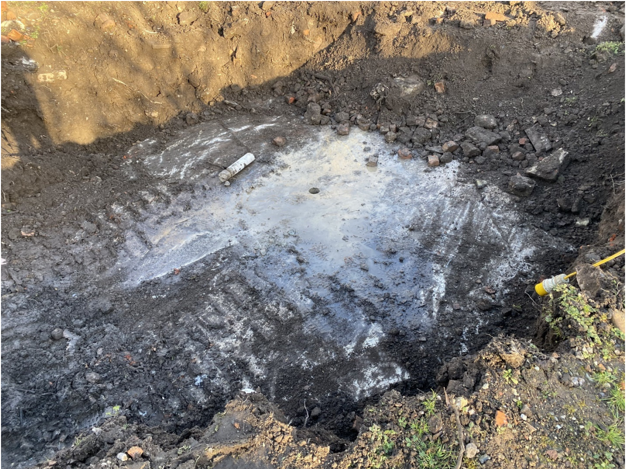
Photograph 3 – Original location of SHAFT 001, before actual location identified
