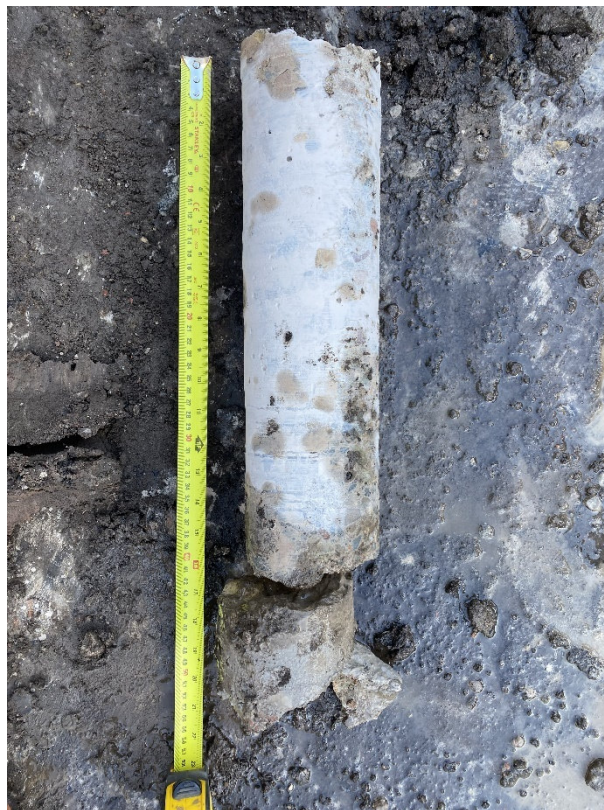
Photograph 4 – Thickness of concrete foundation cored
