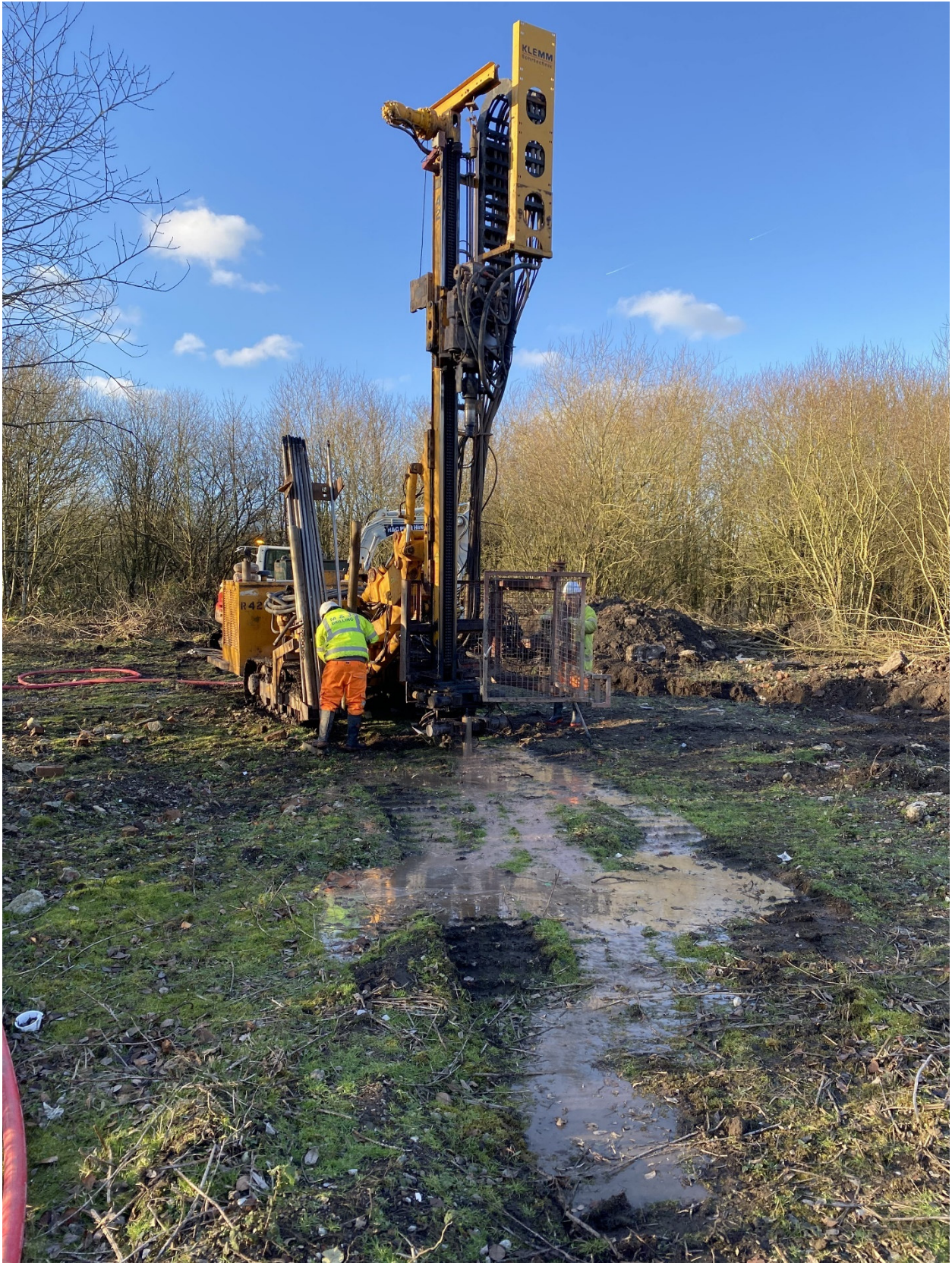
Photograph 1 – Probe drilling of linear lines
