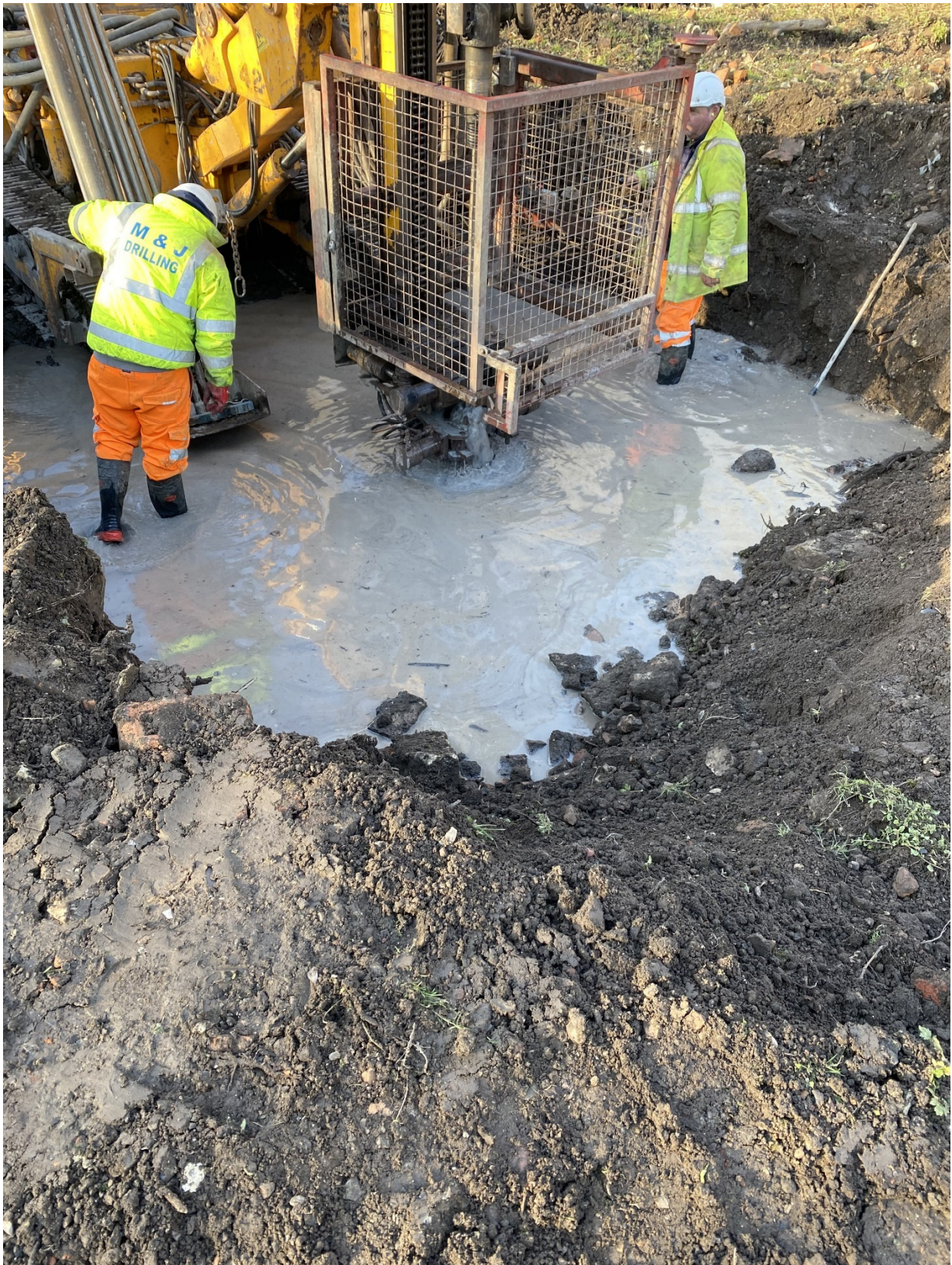
Photograph 2 – investigation of SHAFT 001
