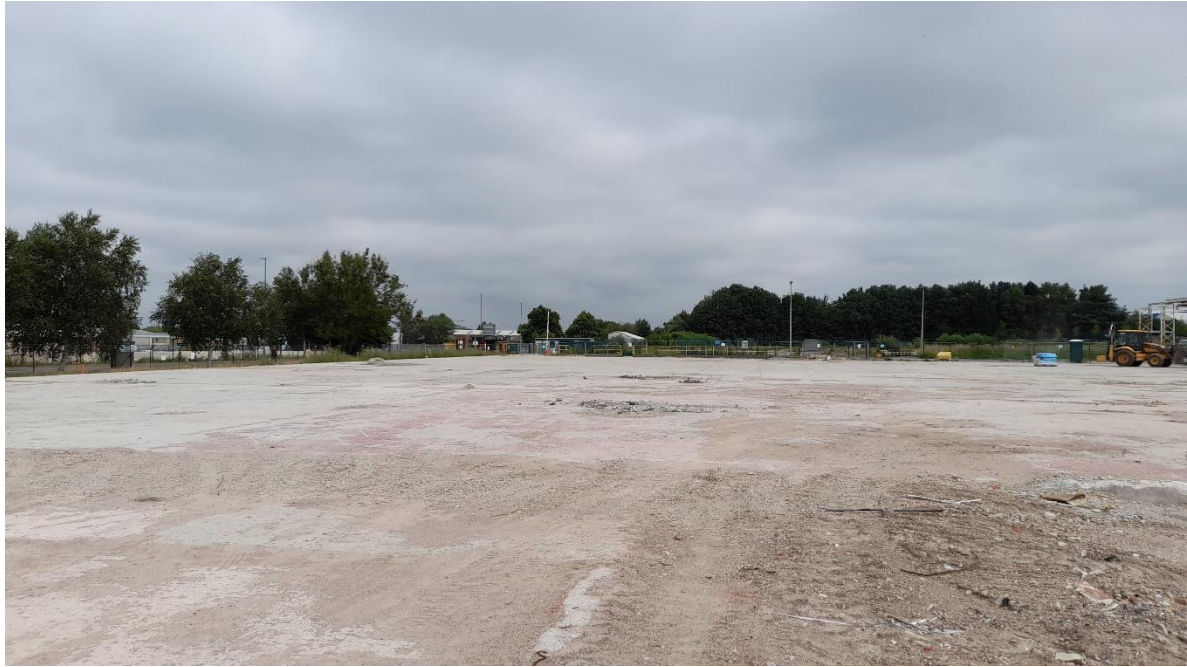
Photograph 56 – Western part of the Site looking north
