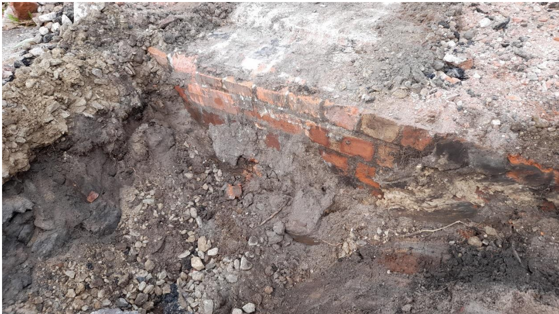
Photograph 24 – TP11 – Brick wall
