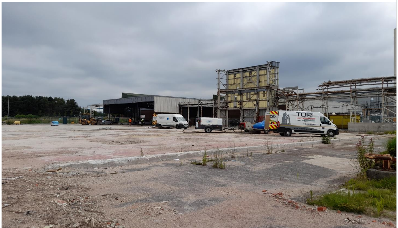
Photograph 57 – Western part of the Site looking north-east
