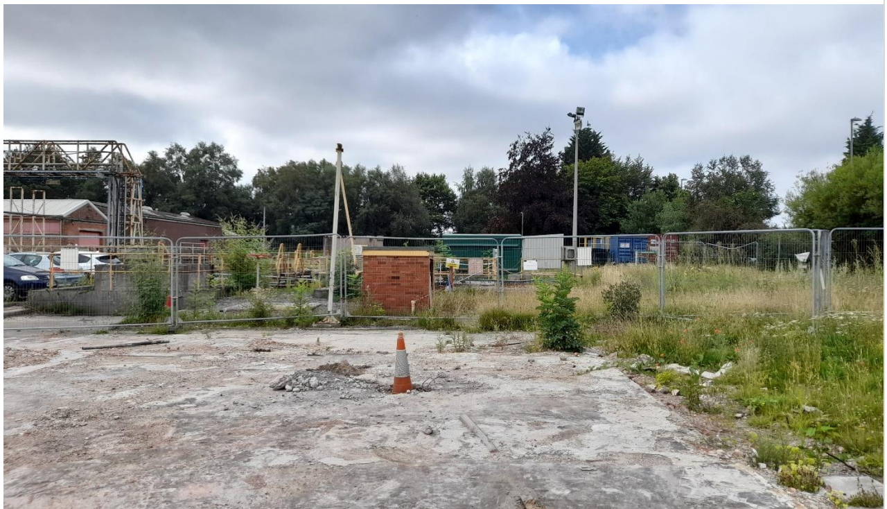
Photograph 61 – Treatment tanks in the south-western corner (beyond fencing)
