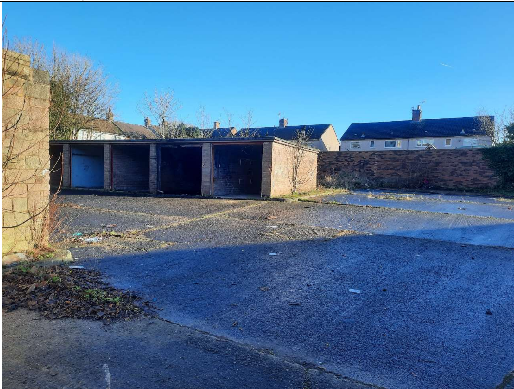
Photo 2 – Showing rows of garages in the south east of the site, taken from the southern site entrance
