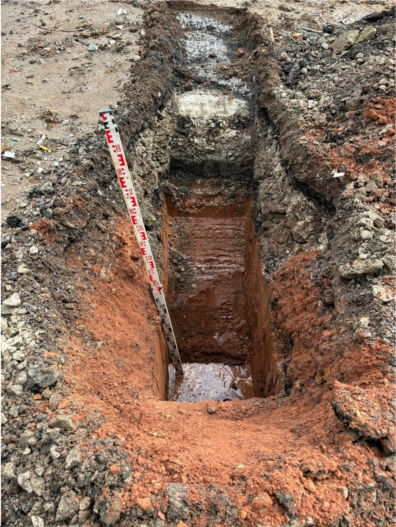
Plate 9: TP09 showing northern face and the concrete at the top of excavation
