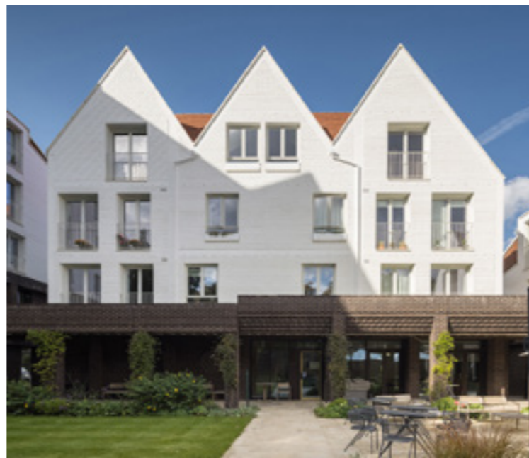
Feature gables: Make a feature out of the gable end to break up the mass of the building
