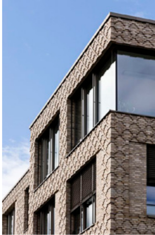
Contextual brick with positive identity: Brick building mass with punched / highlighted windows that are framed by a contrasting material
