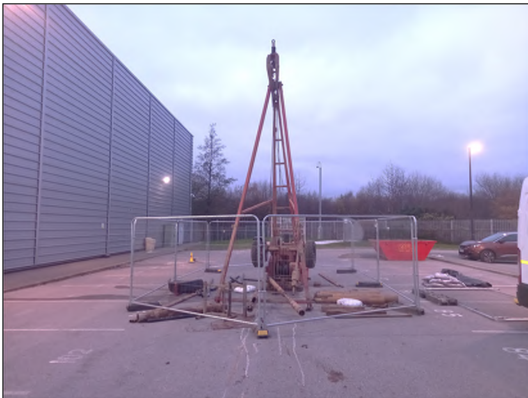
Photo Plate No. 06: Dando 2000 cable pit rig at location CP01, facing south.
