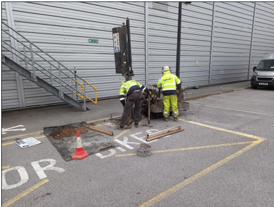
Photo Plate No. 03: Earth Engineering sub-contractors with tracked windowless sampling rig at location WS01.
