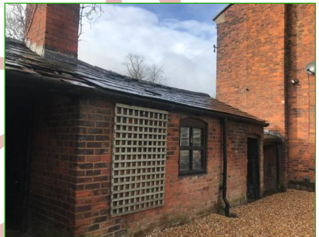
The northeast elevation of the outbuilding
