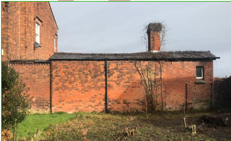
The southwest elevation of the outbuilding
