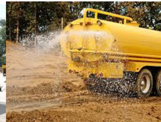
Figure 15. Dust Suppression
