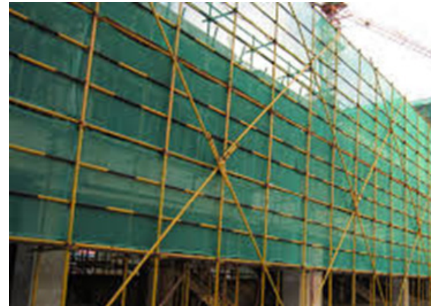
Figure 12. Debris netting
