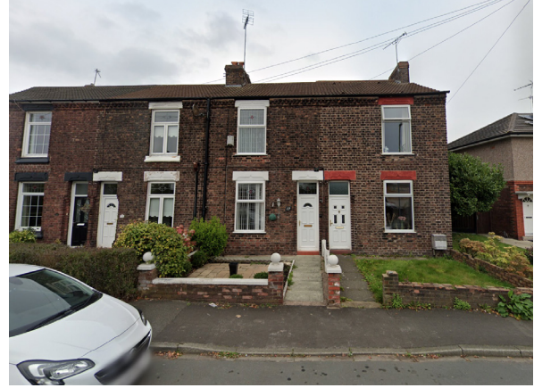
02 - Old Terrace, Hall Lane
