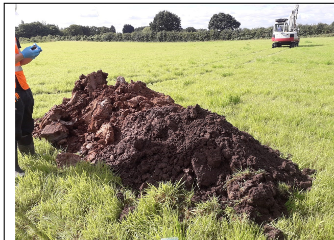
Trial Pit 104/ Soakaway 102 Spoil
