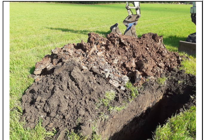
Trial Pit 117 Spoil
