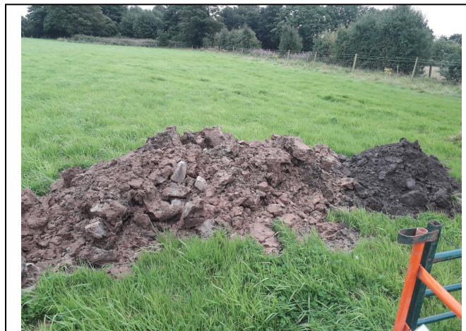
Trial Pit 106/ Soakaway 104 Spoil
