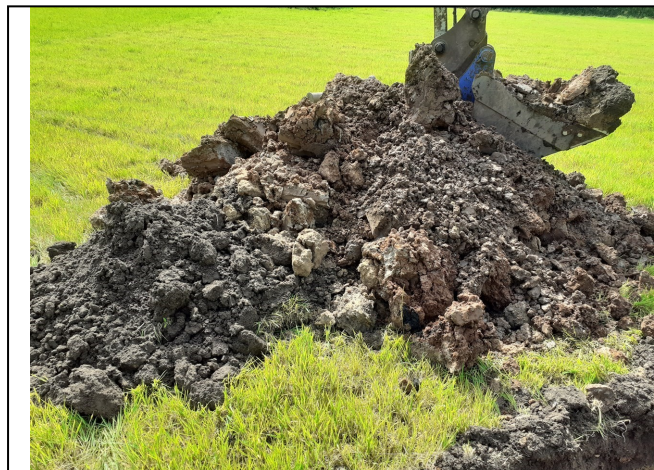
Trial Pit 113 Spoil
