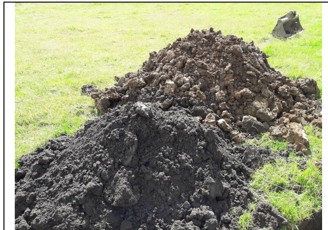
Trial Pit 139 Spoil
