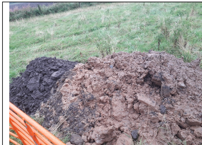
Trial Pit 105/ Soakaway 103 Spoil
