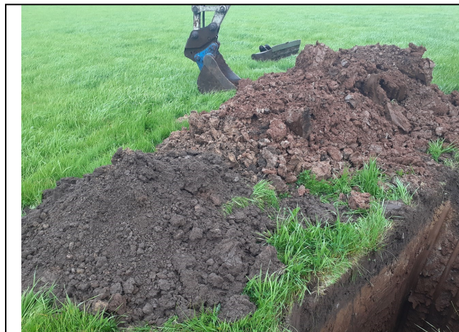
Trial Pit 120 Spoil
