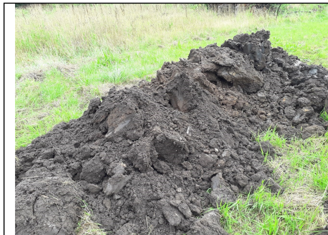
Trial Pit 133 Spoil
