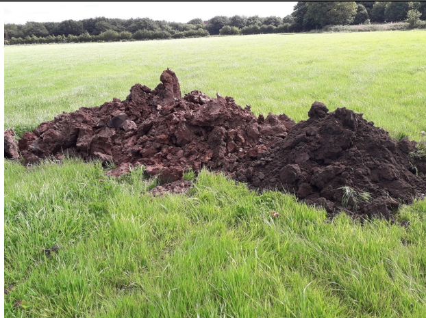
Trial Pit 107/ Soakaway 105 Spoil
