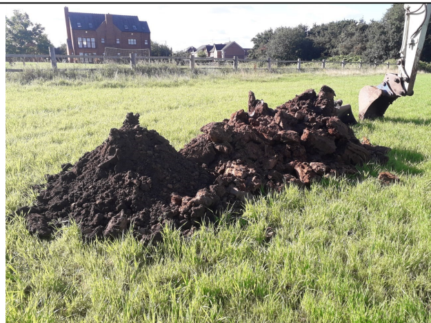
Trial Pit 101/ Soakaway 101 Spoil
