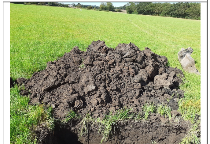
Trial Pit 116 Spoil
