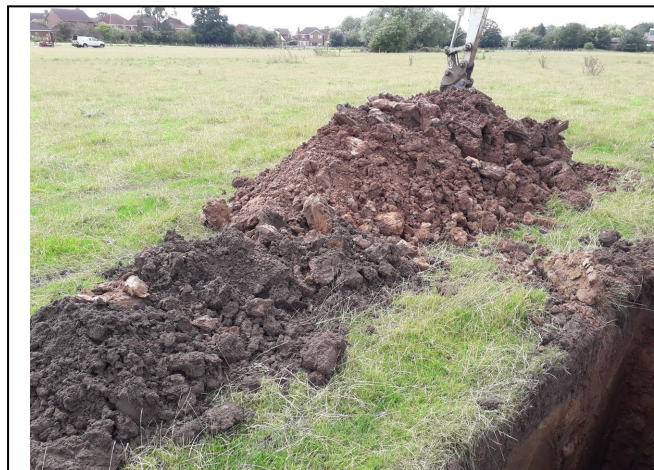
Trial Pit 138 Spoil
