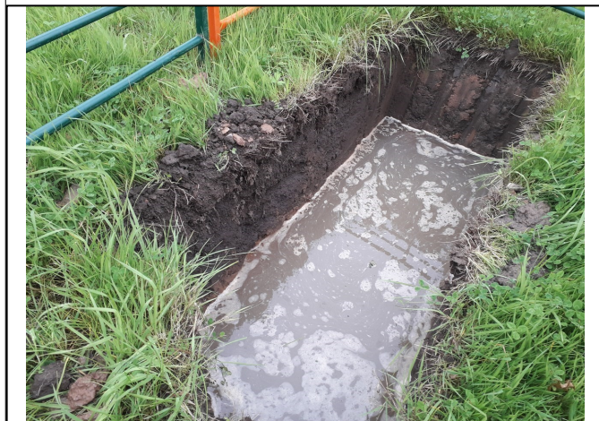
Trial Pit 106/ Soakaway 104
