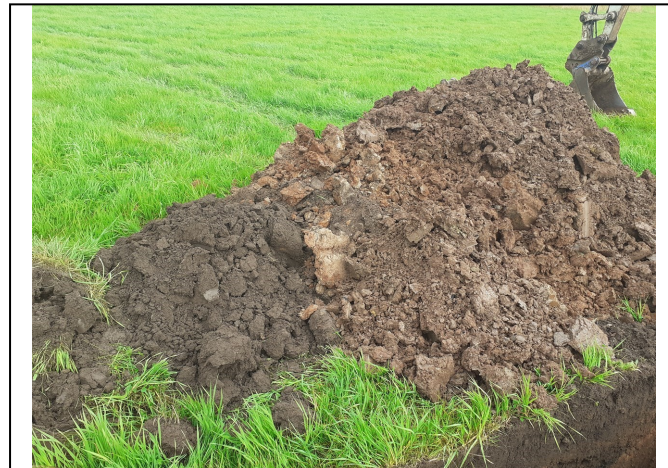
Trial Pit 124 Spoil
