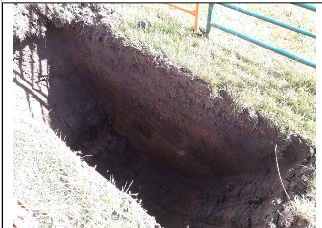
Trial Pit 108/ Soakaway 106
