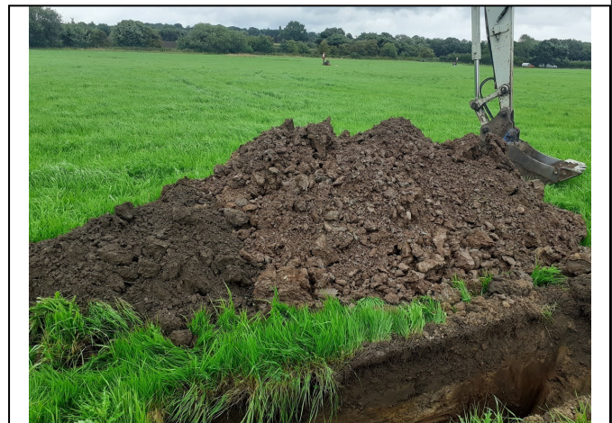
Trial Pit 127 Spoil
