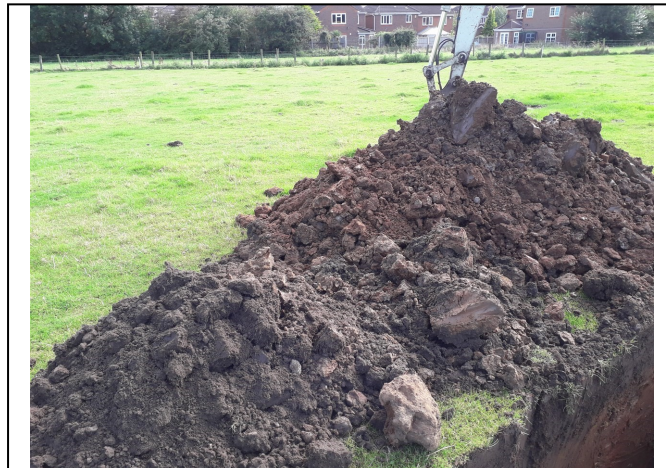
Trial Pit 142 Spoil
