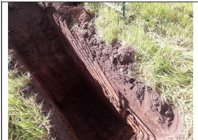
Trial Pit 104/ Soakaway 102
