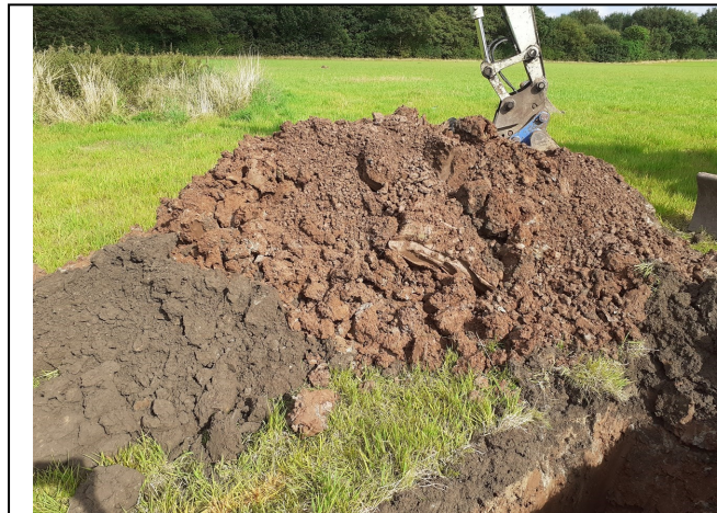
Trial Pit 118 Spoil
