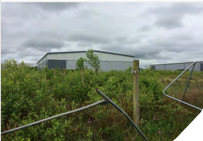
Photo 11: Heras fencing on site, separating the north and south portion of the site
