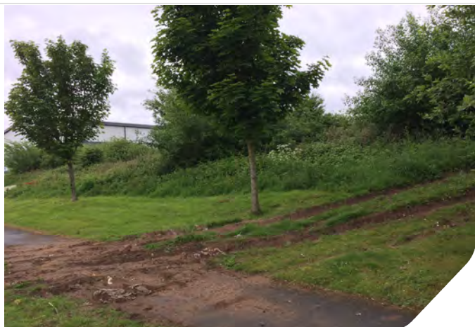
Photo 02: Vegetation bund along the eastern site boundary, showing evidence of vehicle access onto site.
