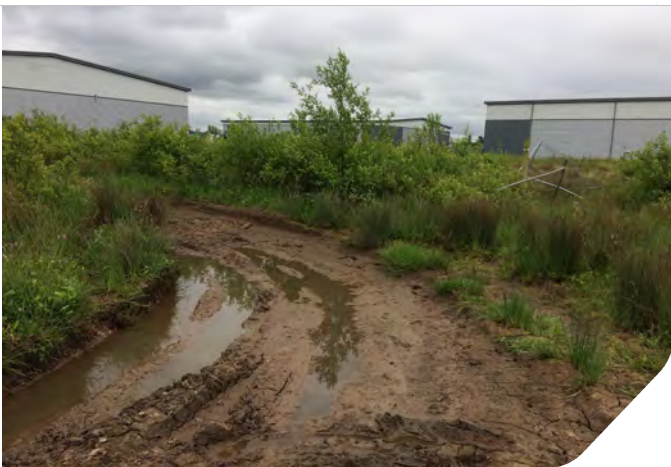
Photo 10: evidence of surface water pooling in the east of the site
