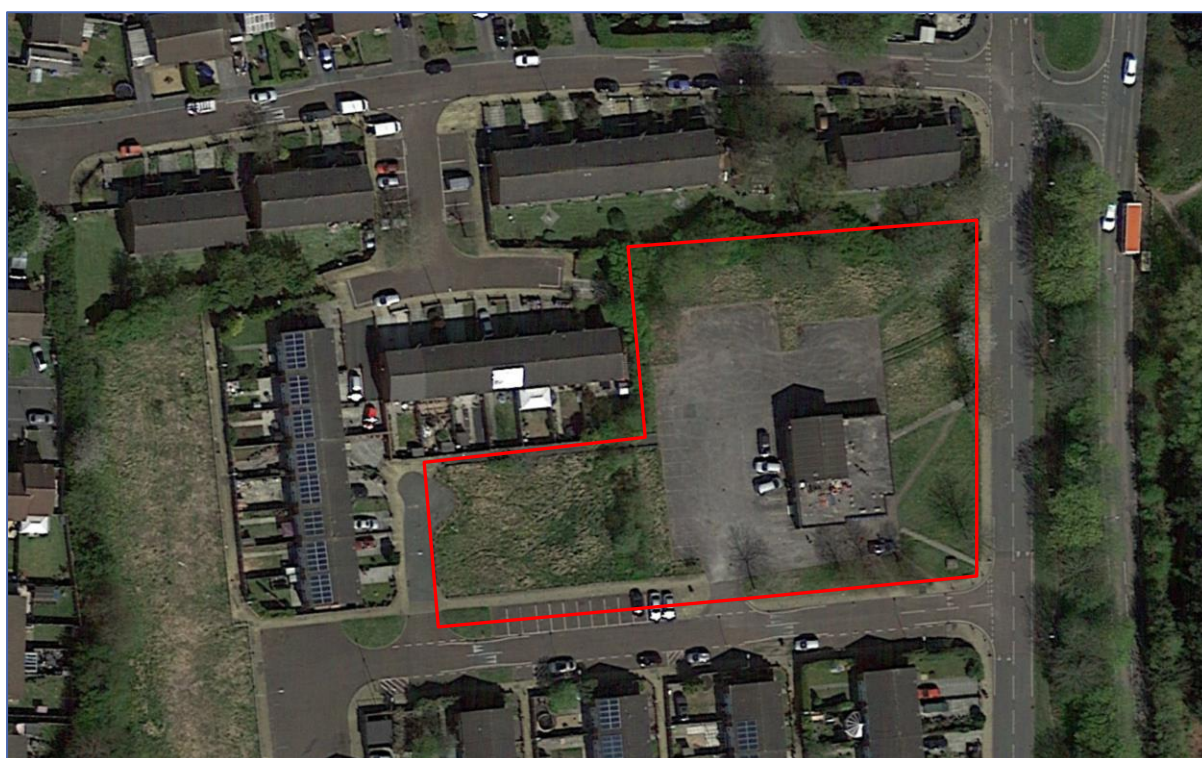
Figure 2 - Aerial view of site (boundary marked in red)
