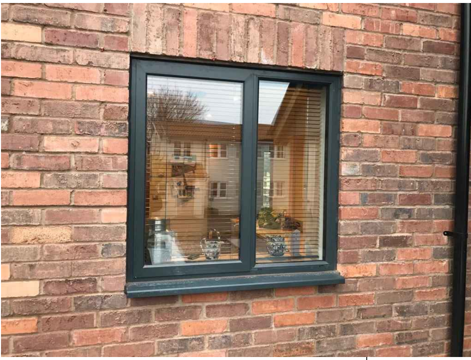
Aluminium Double Glazed Windows (RAL 7016 - Dark Grey)
