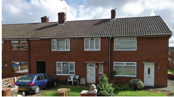
Fisher Avenue - Terraced Properties
