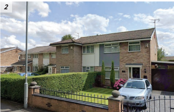
Driveway - Semi-Detached Properties
