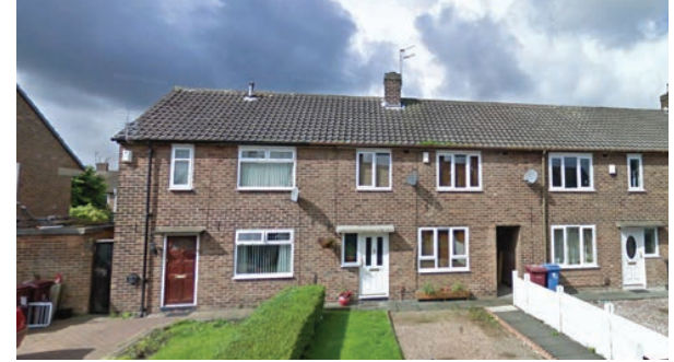
Fisher Avenue - Terraced Properties
