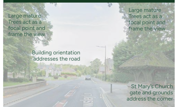
St Mary's Church Approach
