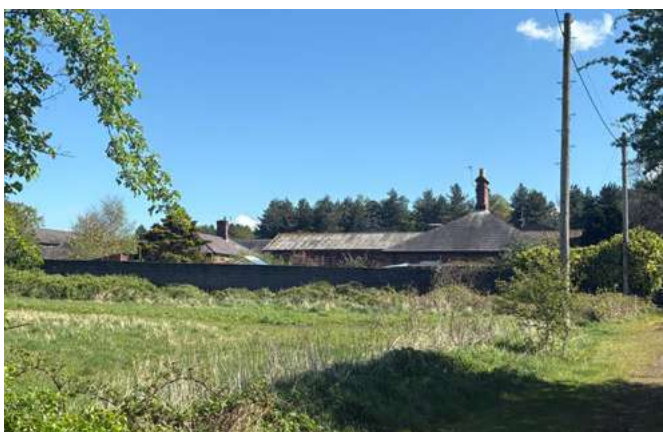
3. Home Farm Lodge (Stanley Grange Business Village)
