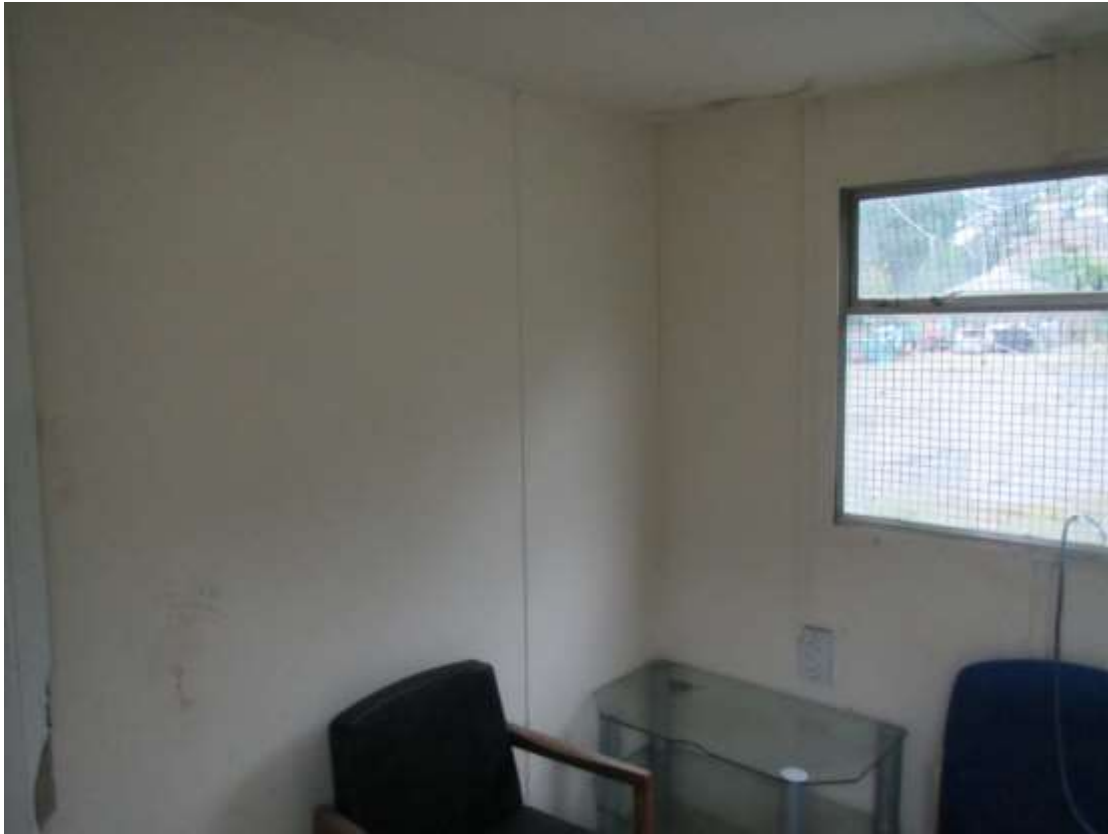
Photograph 15 – Inside of Building 3.
