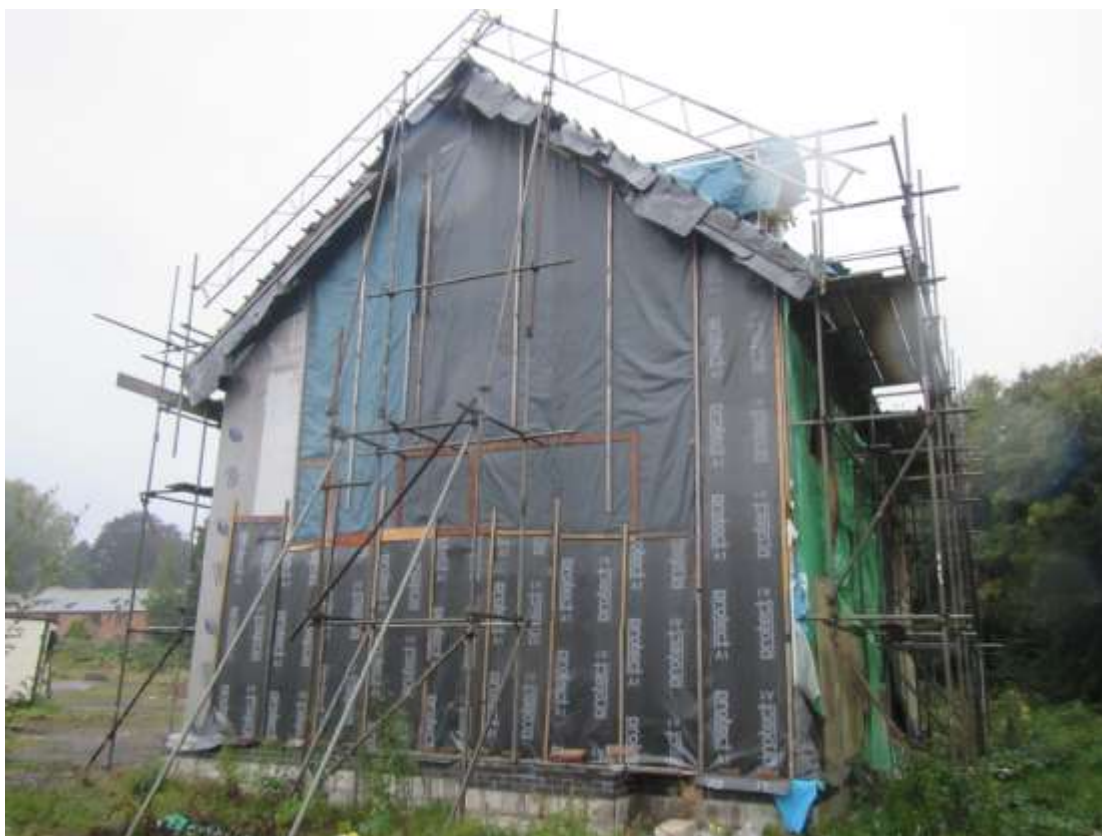
Photograph 3 – The south-eastern aspect of Building 1.
