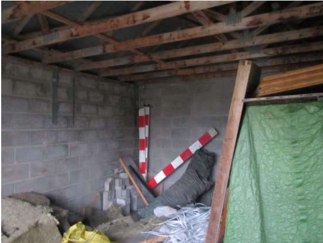
Photograph 13 – Internal view of Building 2.
