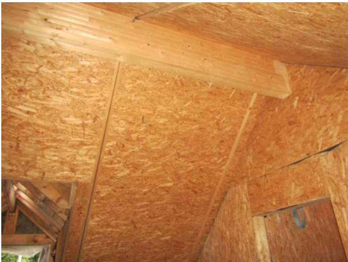
Photograph 10 – Looking at the underside of roof within Building 1.
