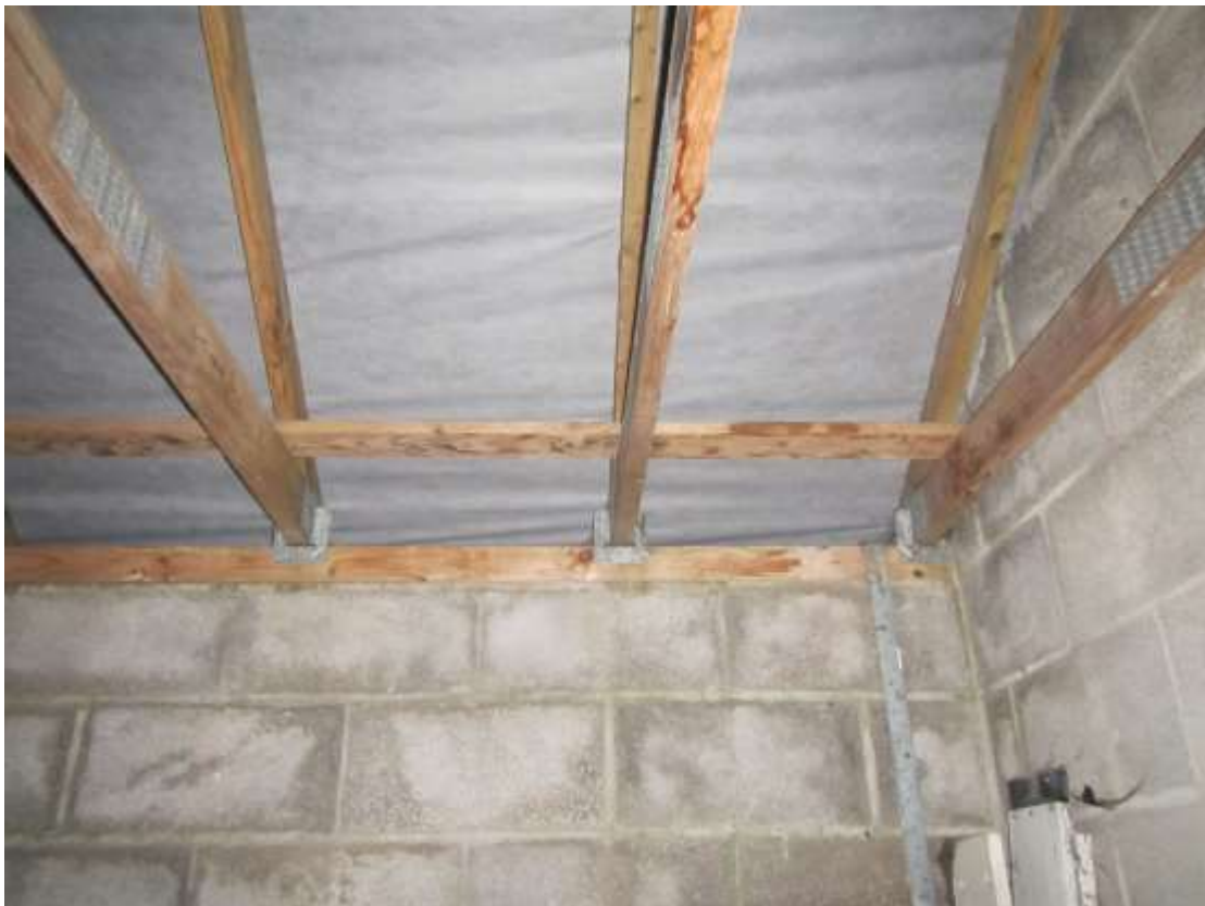
Photograph 14 – Showing the roof lining of Building 2.
