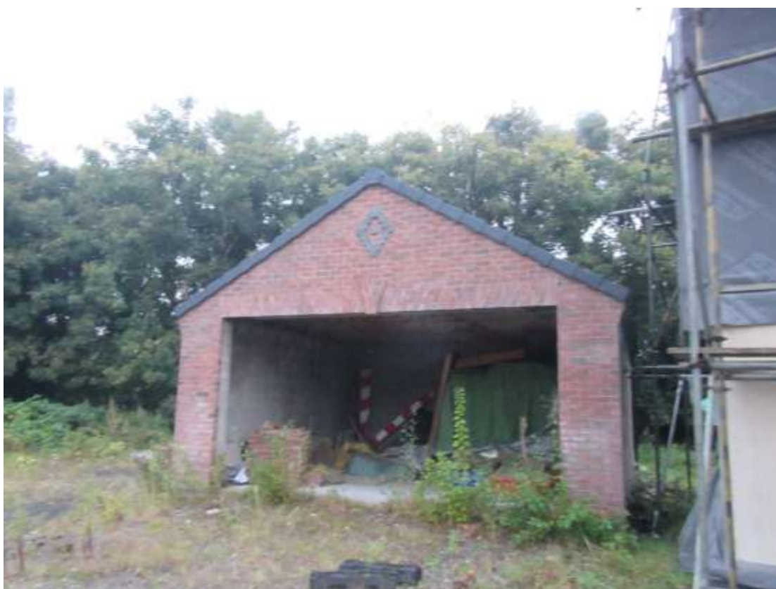
Photograph 4 – The south-western aspect of Building 2.
