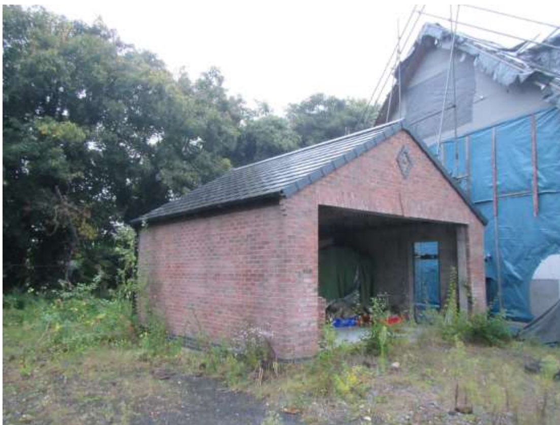
Photograph 5 – The north-western and south-western aspect of Building 2.
