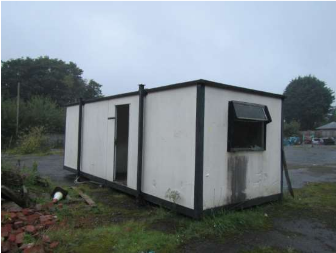
Photograph 7 – The north-western and north-eastern aspect of Building 3.
