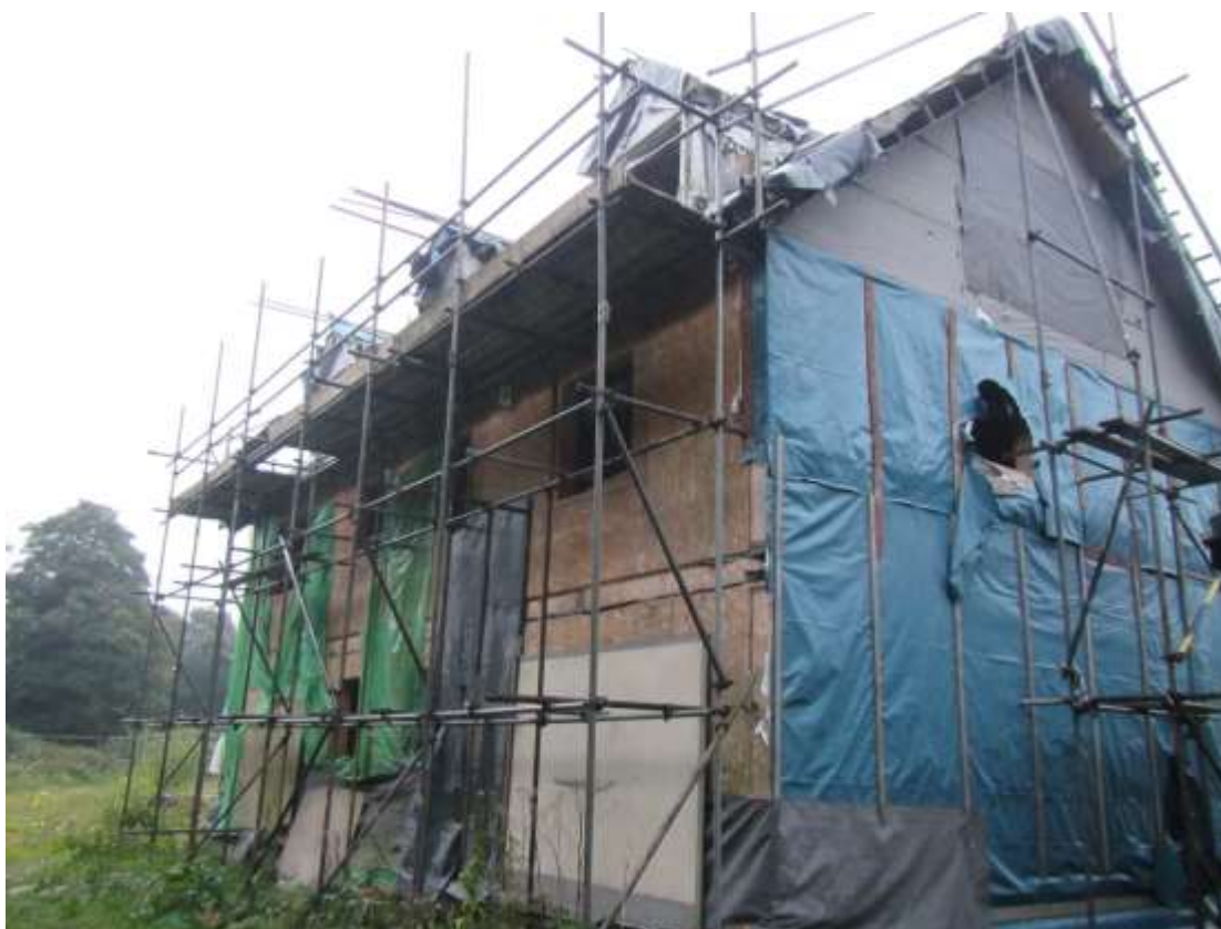
Photograph 2 – The north-eastern and north-western aspect of Building 1.
