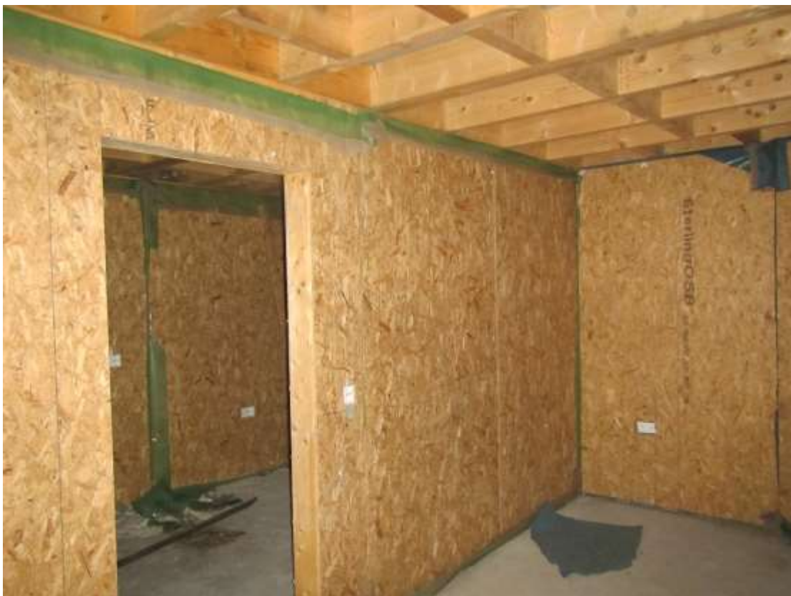
Photograph 8 – Internal area of Building 1.
