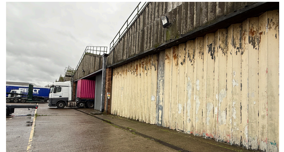
Tired/dated existing warehouse building on site
