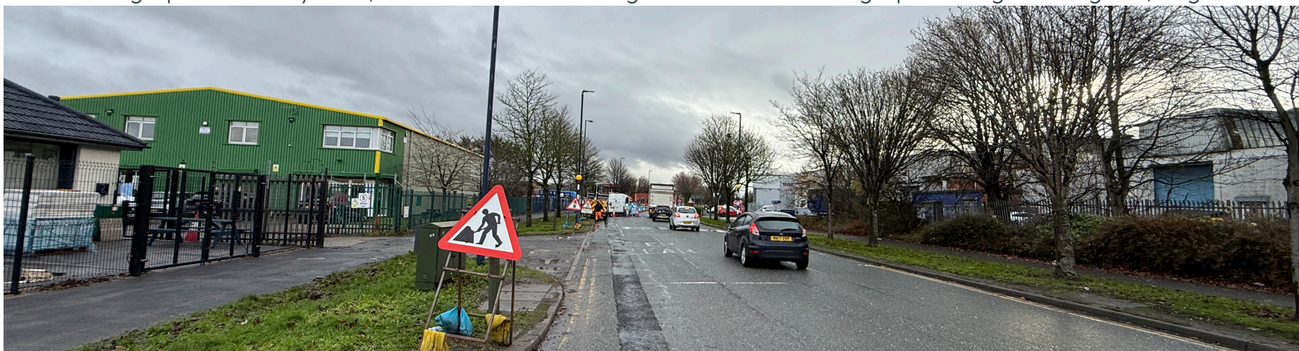
Photograph looking southeast down Wilson Road, industrial units fronting the highway
