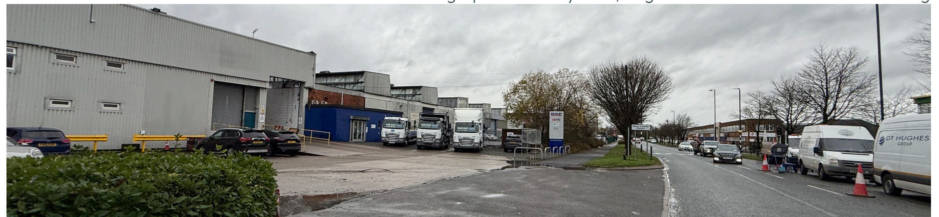
Photograph of site adjacent, large units with extensive hard standing
