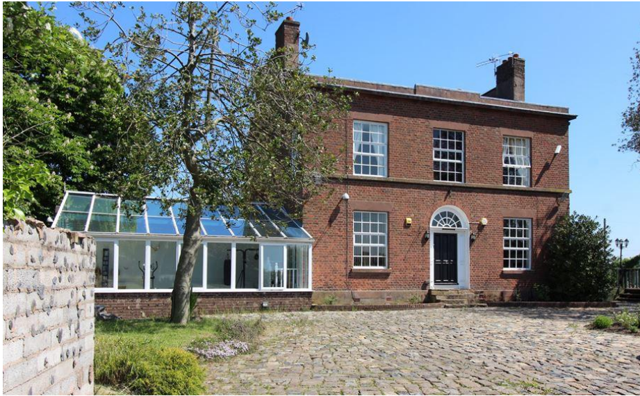
Figure 2: Image showing the front of the property
