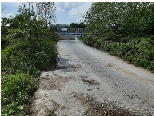
Photograph 3: Western access into the Site from Coopers Lane (U3).
