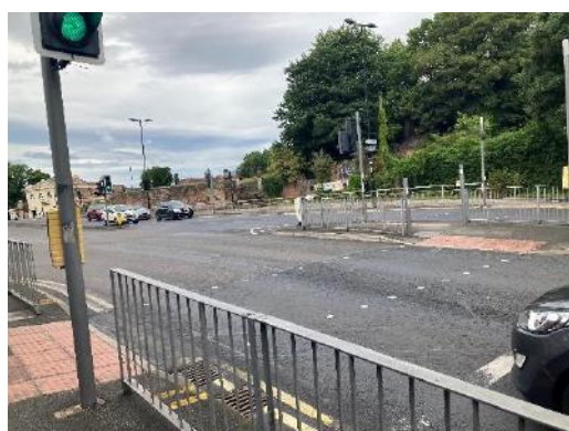
Photograph 9: Pedestrian Signalised Crossing at Huyton Lane viewing westbound
