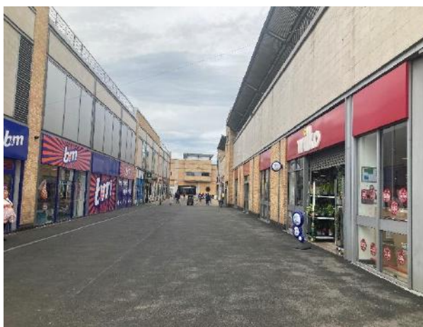
Photograph 13: Pedestrian Conditions within Huyton town centre
