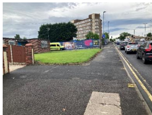
Photograph 4: Site frontage conditions viewing westbound
