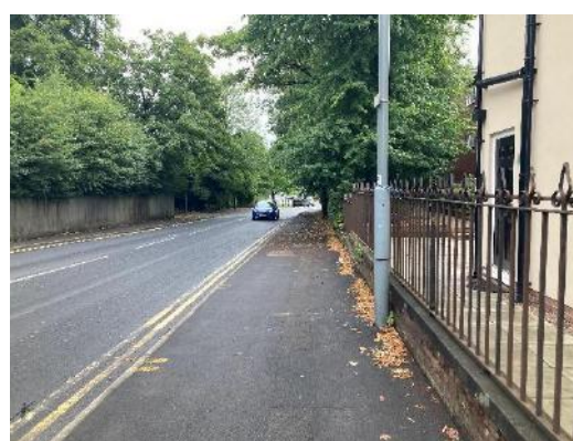
Photograph 6: Pedestrian footway conditions headed eastbound along Huyton Lane
