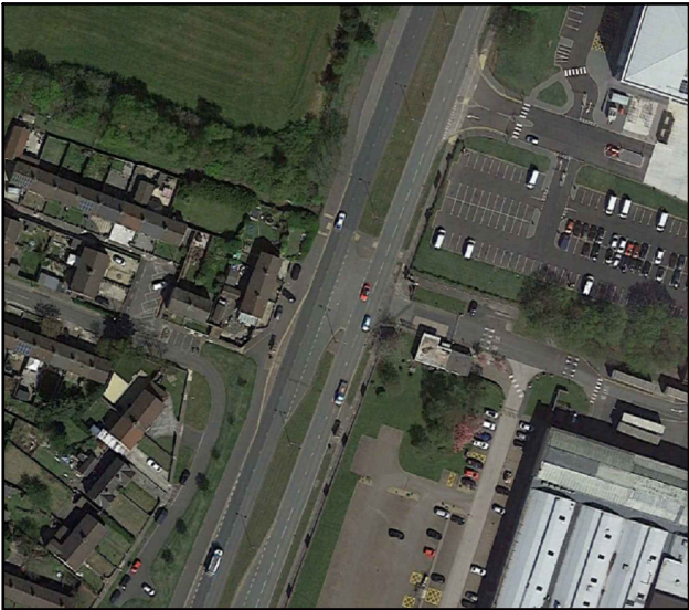
NORTH SOUTH AERIAL VIEW
