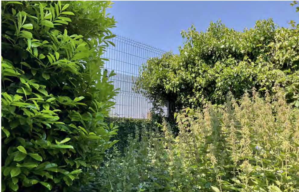
9. View of existing metal mesh fence. Upper mesh fence to be removed.
