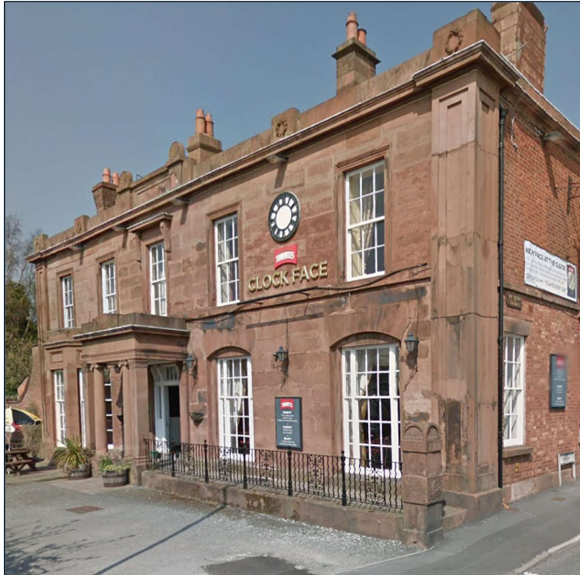
Plate 5 – April 2015: Existing building mounted sign and amenity board sign installed by this date.
