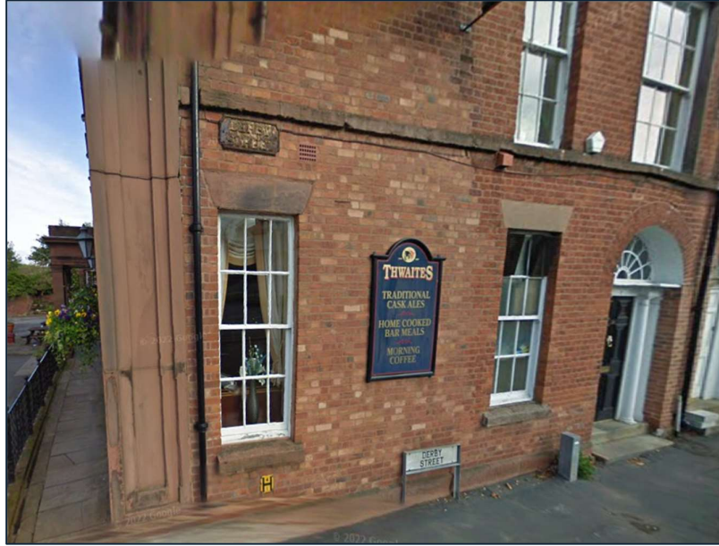
Plate 1 – September 2011: Previously installed amenity board to the southeast elevation.
