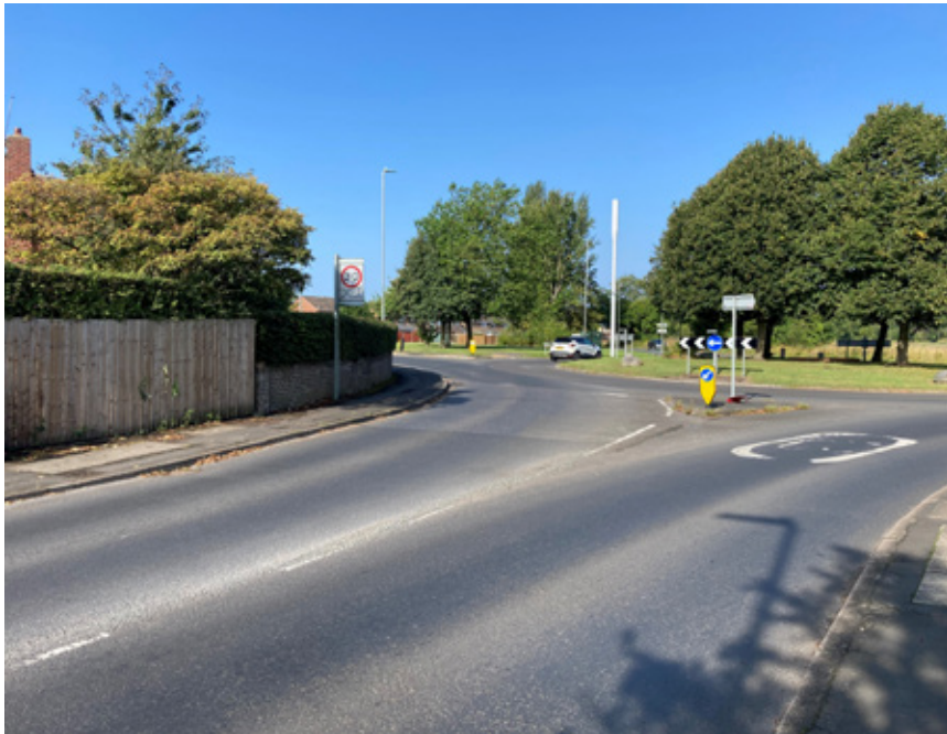
Church Road (east) – footpath on the east bound side
