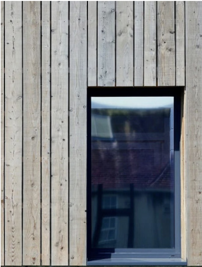
Flat Timber Cladding - Tongue and Groove
