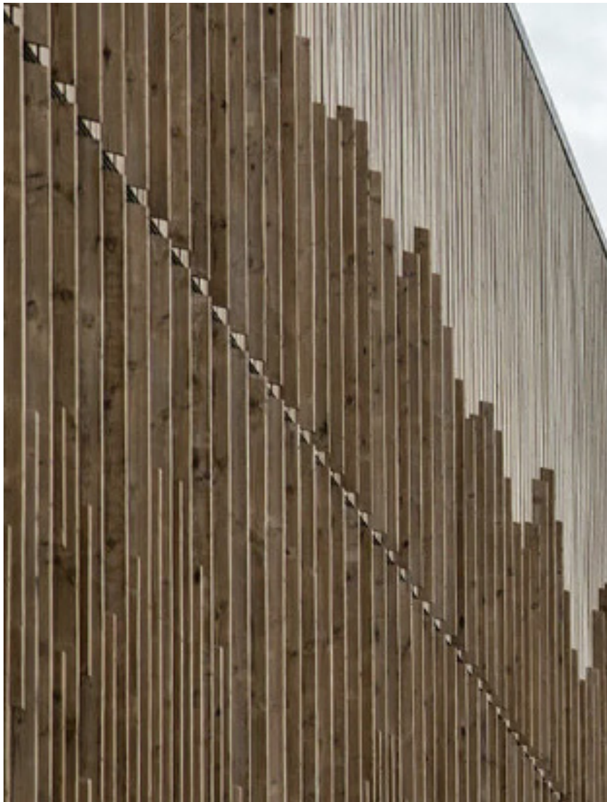
Vertical Patterned Timber Cladding
