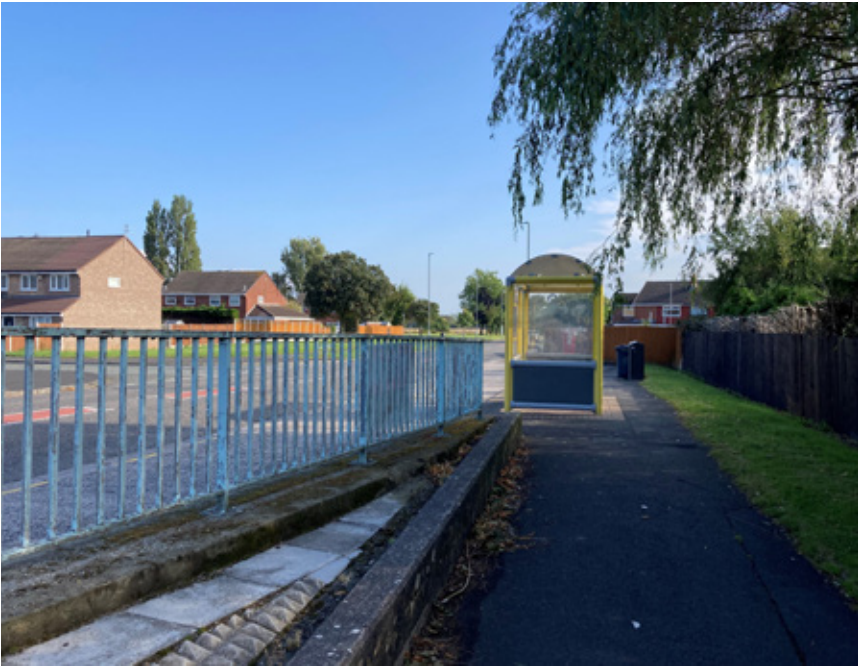
Okell Drive – footpath on south-west bound side
