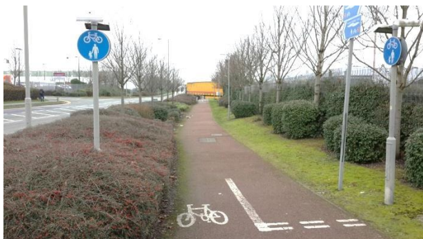
Figure 5.28: TPT route section on the western perimeter road
