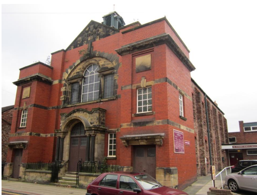
Prescot Wesley Methodist Church (unaffected by the proposed work at 19 Atherton Street)
