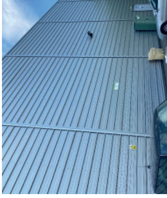
Existing Ventilation Louvre
