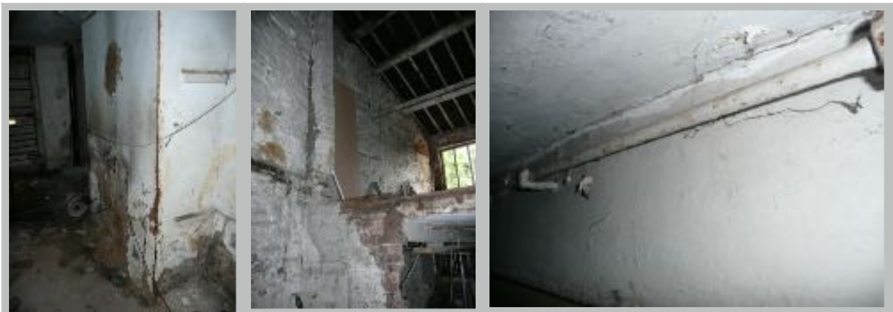
Plate 16. Chimney piece at E end of Brewery House
