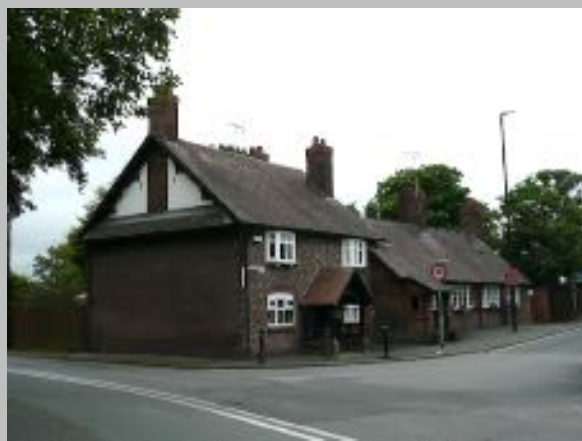
Plate 30. Former Post Office
