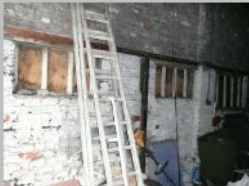
Plate 11. Internal face of S wall of the stables/barn
