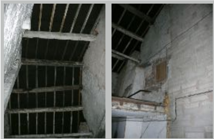
Plate 14. Purlins and ridge at E end of Brewery House
