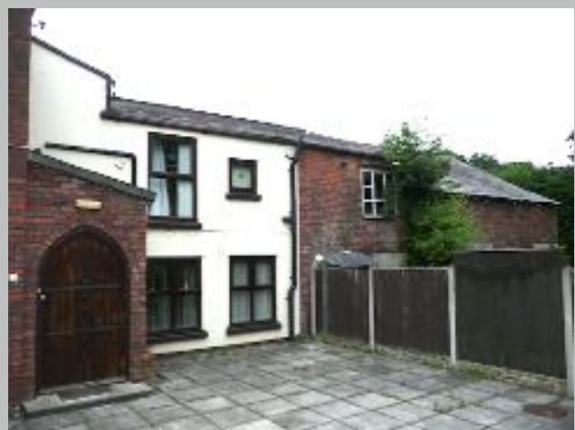
Plate 24. S elevation of Spencer House
