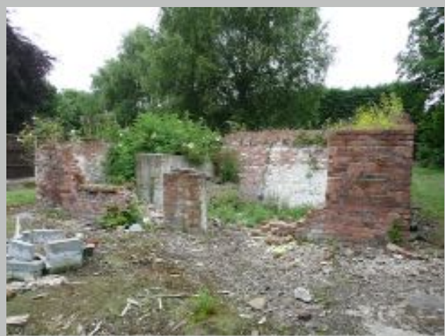
Plate 22. S elevation of detached out building
