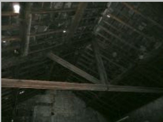
Plate 12. Sawn pine king-post truss
