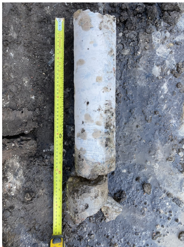
Photograph 4 – Thickness of concrete foundation cored
