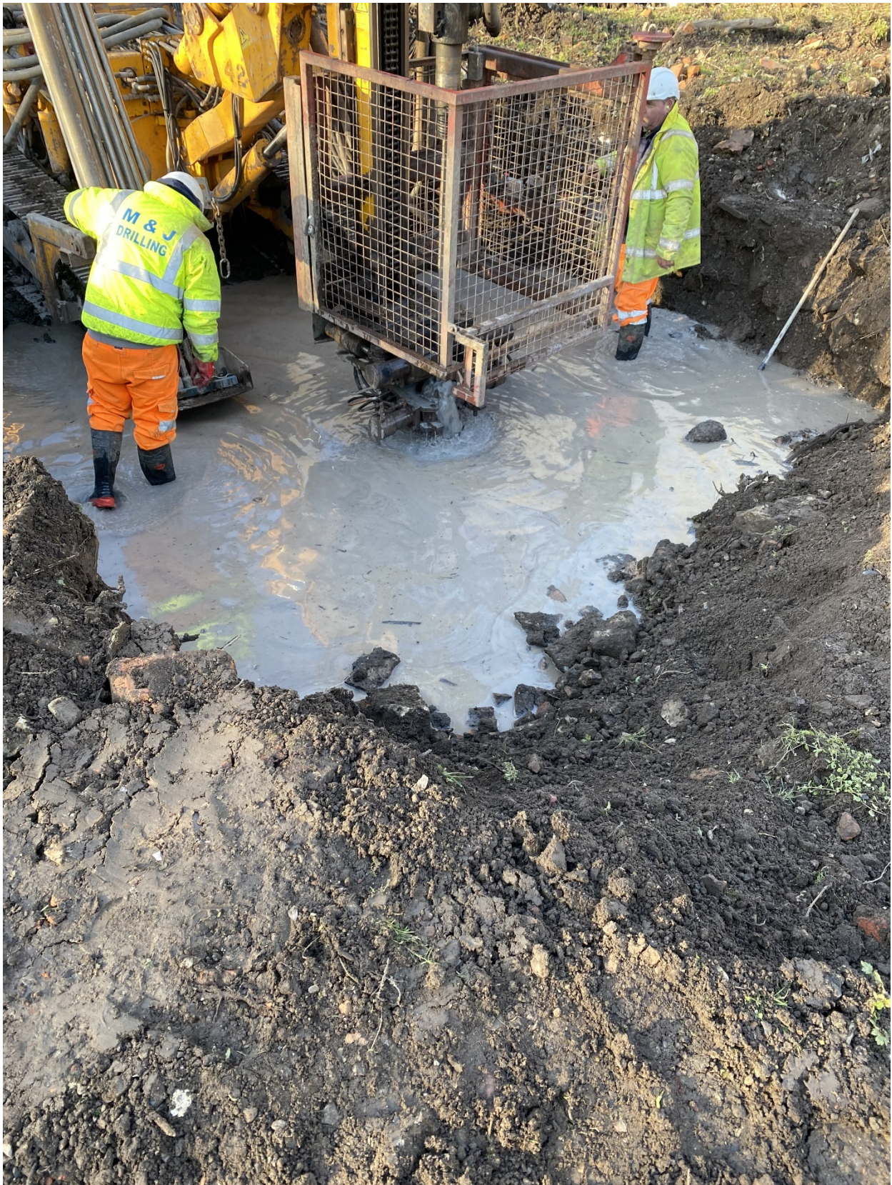
Photograph 2 – investigation of SHAFT 001
