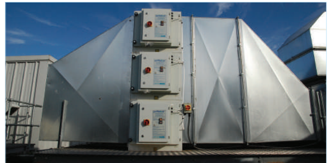
3 ESP Units Stacked in modular formation
