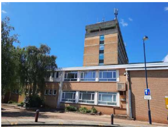
Plate 4.6: Section 1 of Building B4 in Foreground, with Section 2 to Rear.
