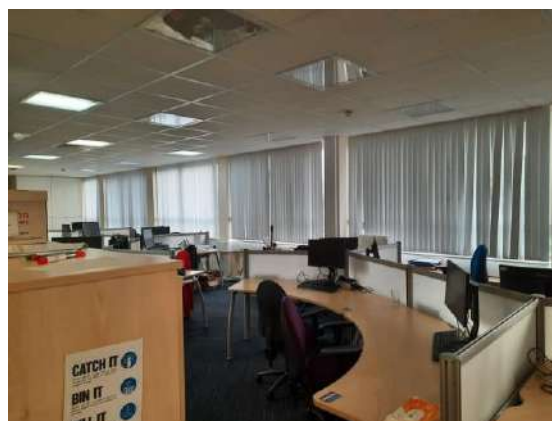
Plate 4.11: Open-plan Office Space on First Floor of Section 2 (Building B4).
