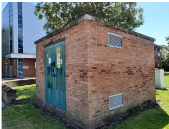
Plate 4.3: North-western and North-eastern Elevations of Building B2.
