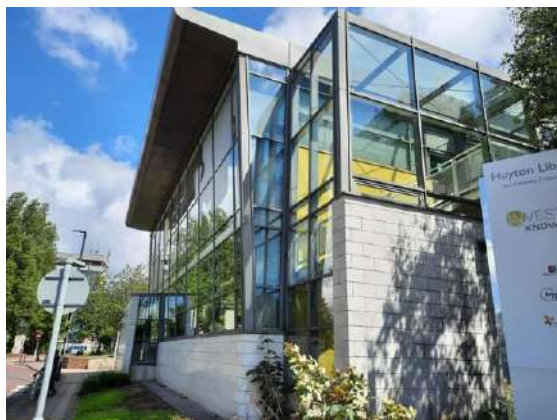
Plate 4.1: Northern Elevation of Building B1.
