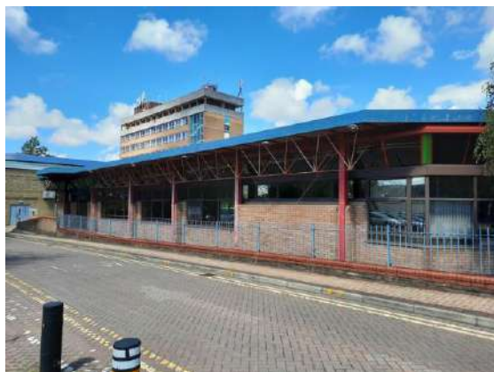
Plate 4.4: Western Elevation of Building B3.
