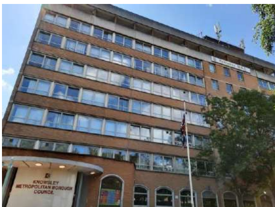
Plate 4.8: North-east Elevation of Section 2 of Building B4.
