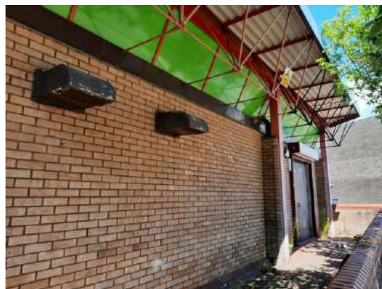
Plate 4.5: South-east Elevation of Building B3, with Vents in Wall and Overhanging Canopy.
