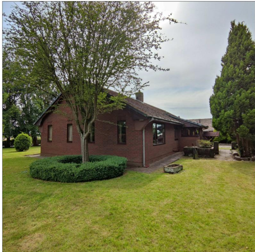
PHOTO 2 - SIDE AND REAR ELEVATION
