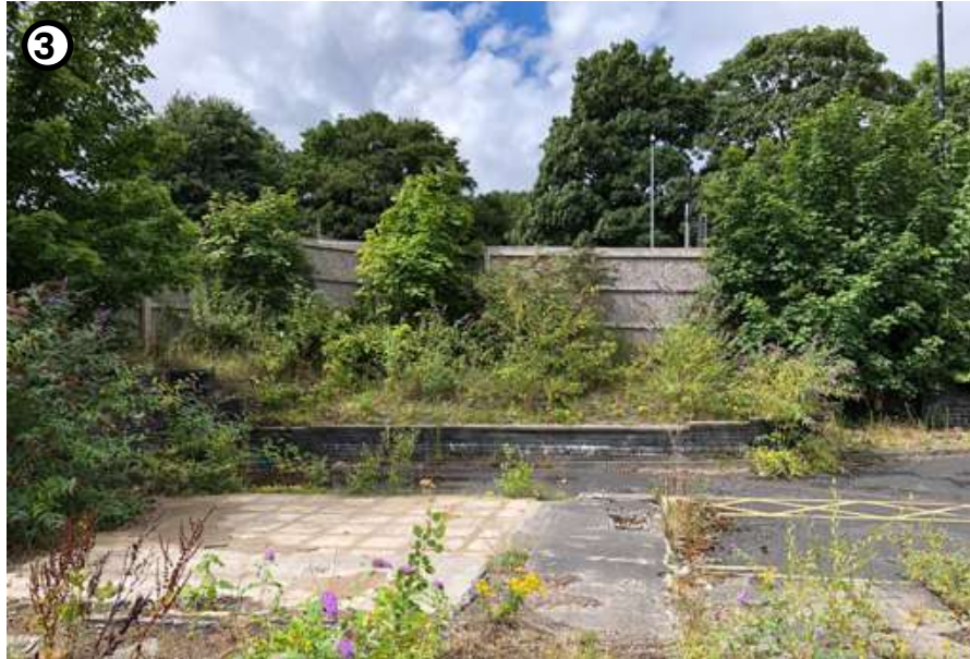
View 3 - View from within site of existing retaining wall in North-West corner.
