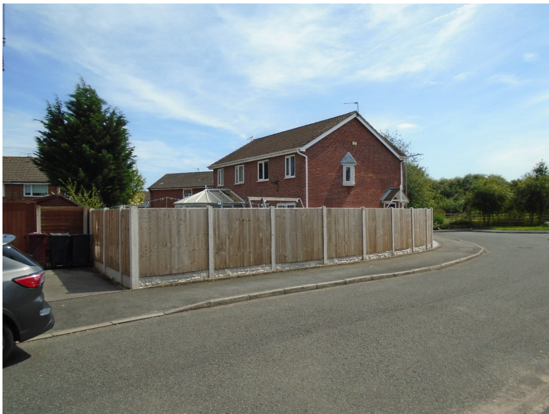
(Photo of Fencing on site)
