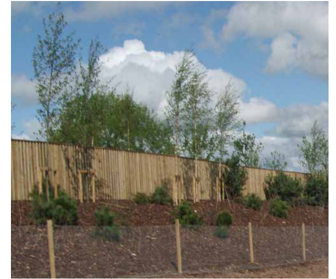
Acoustic fence on a perimeter mound
