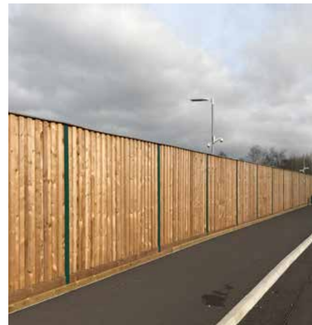
Typical Acoustic Fence
