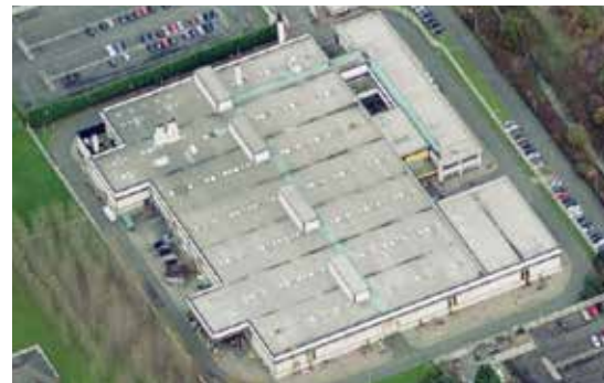
06. Interchange Motorway Industrial Estate
