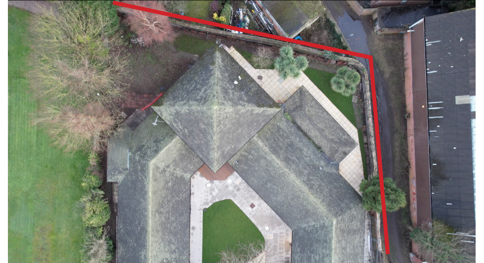
View from above at the North of Plot 11a
