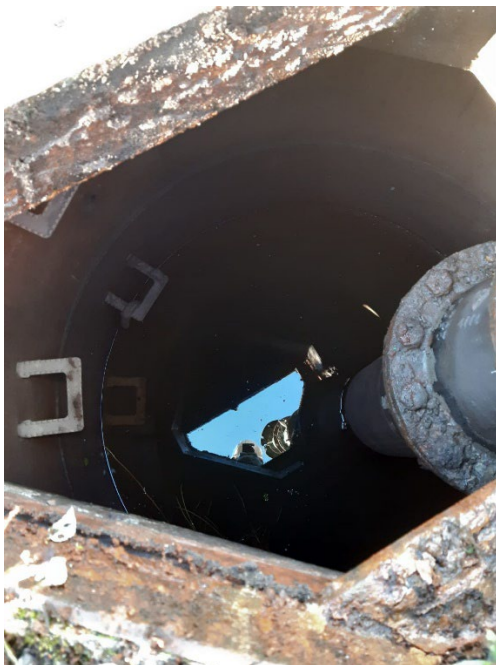
Photograph 3.1. Vent pipe from Shaft No. 1 within inspection chamber (manhole rings).
