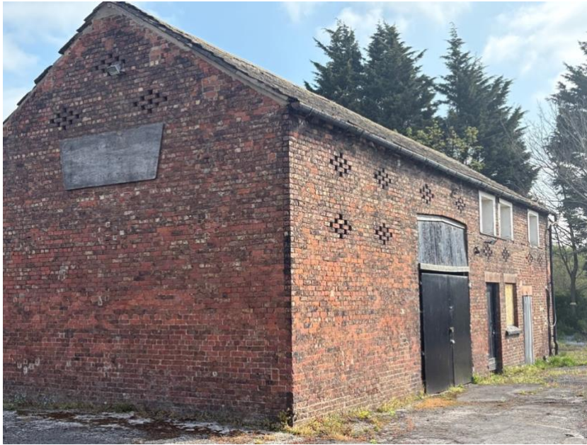
Figure 10- barn- western gable and southern elevation
