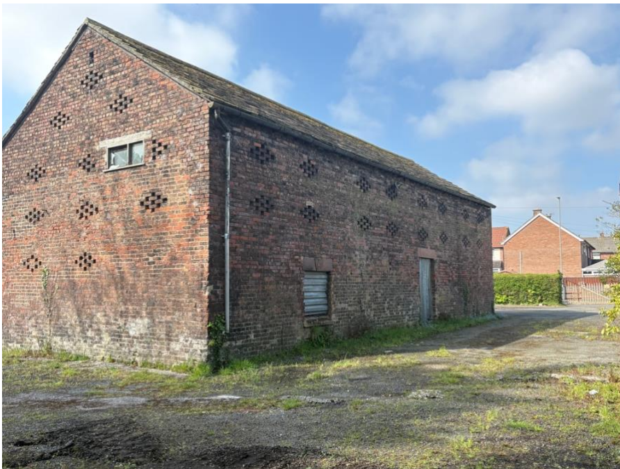
Figure 9- barn, eastern gable and northern elevation
