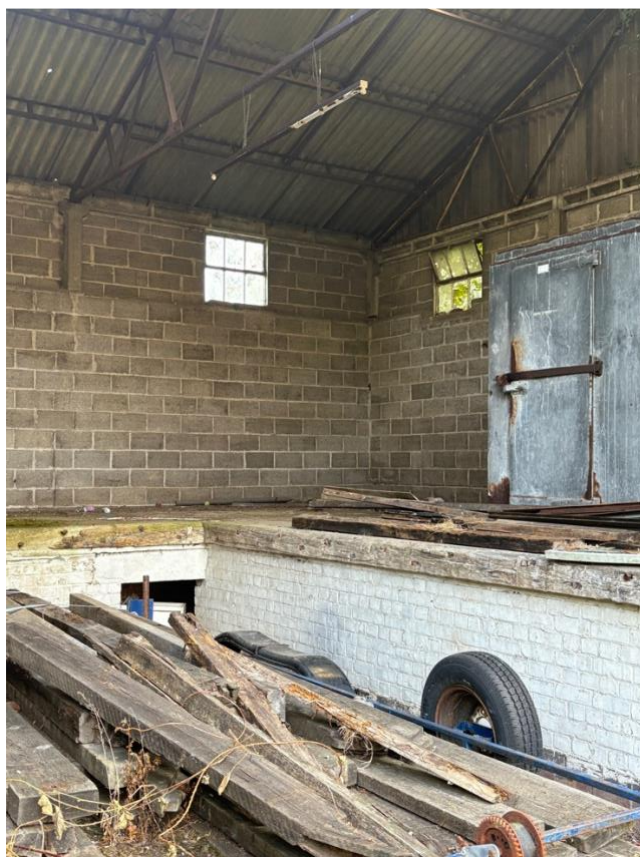
Figure 7- second barn, interior, showing block construction and metal roof trusses
