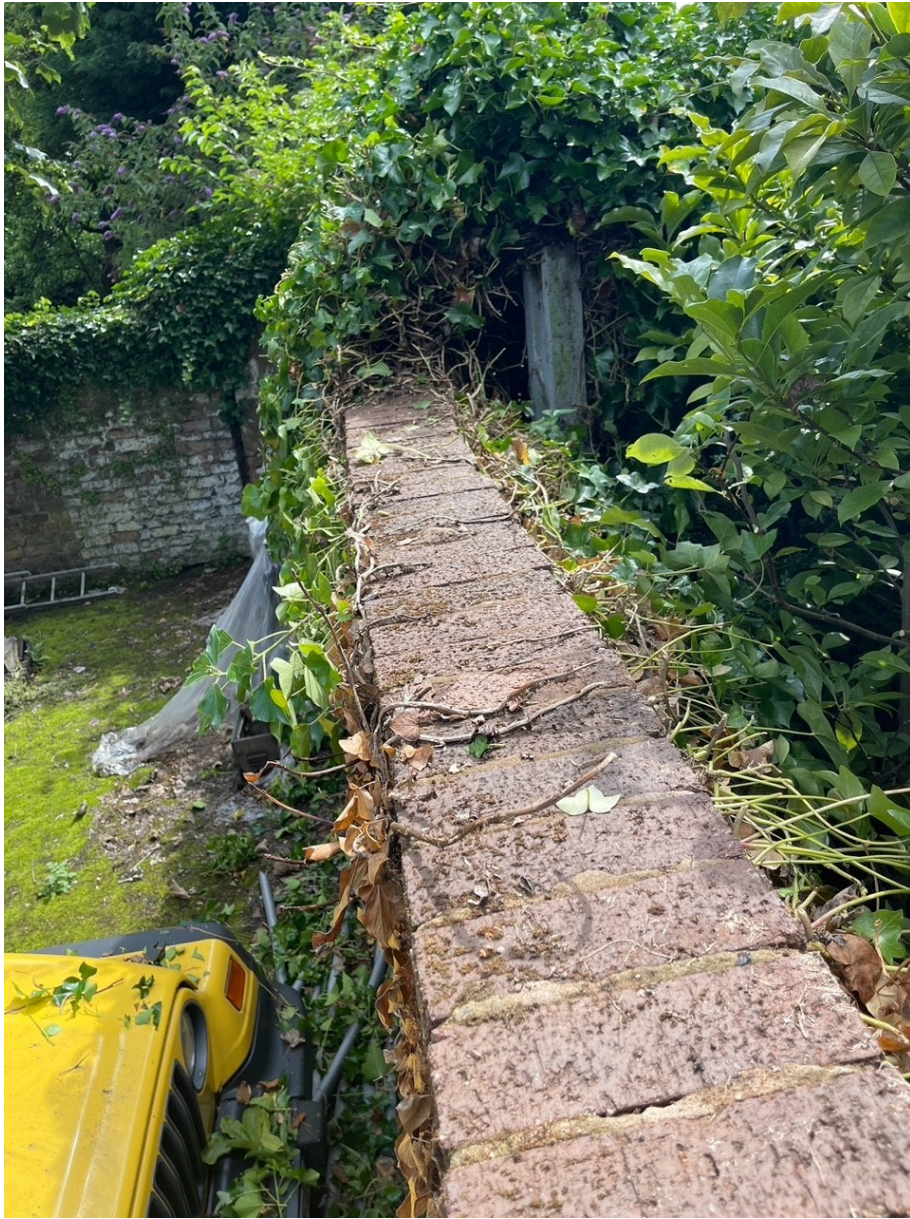
Aerial view of wall looking south (no step in the alignment of the wall)
