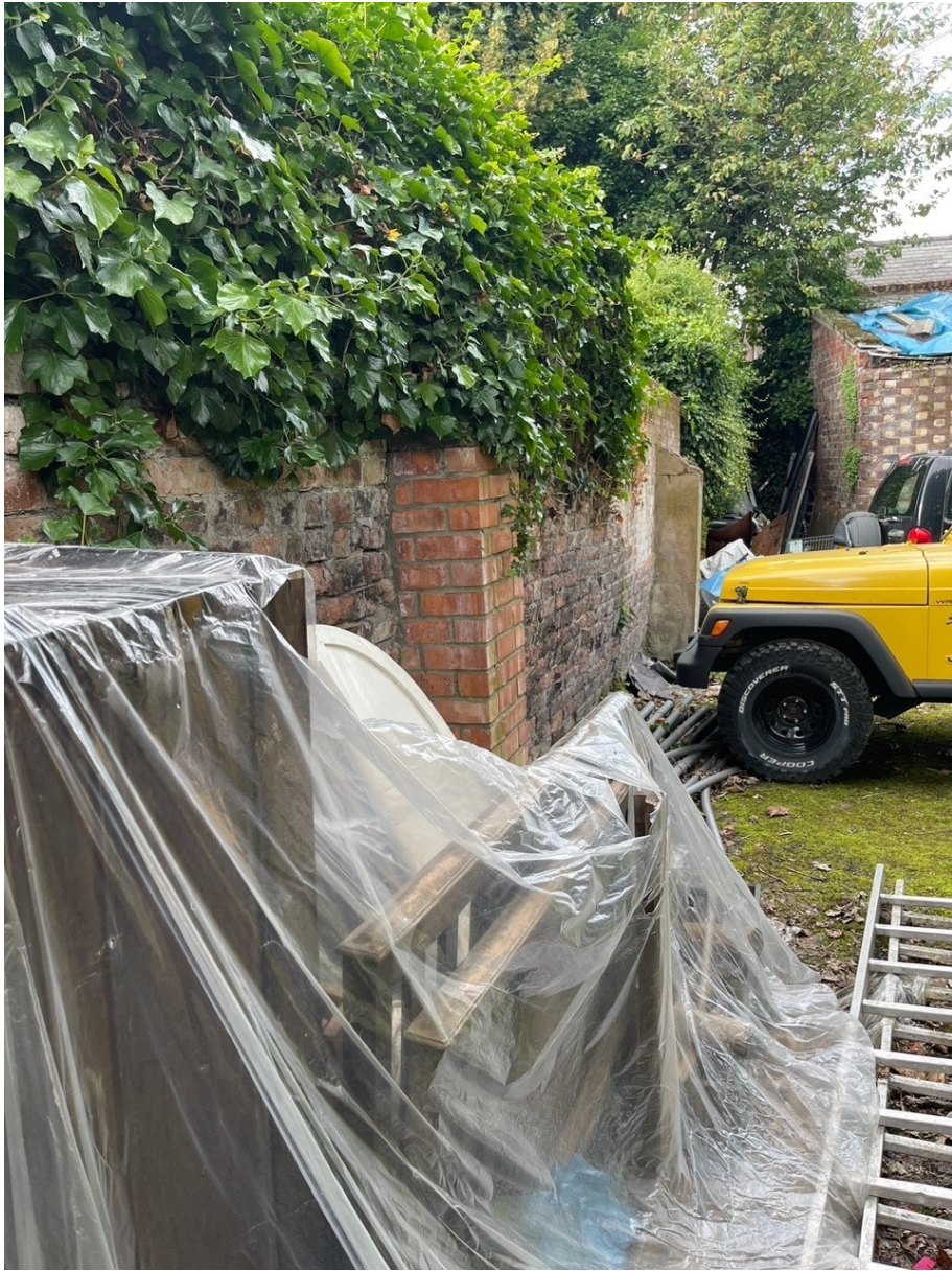
Boundary wall view looking north (no step in the wall at the location of the two buttresses)
