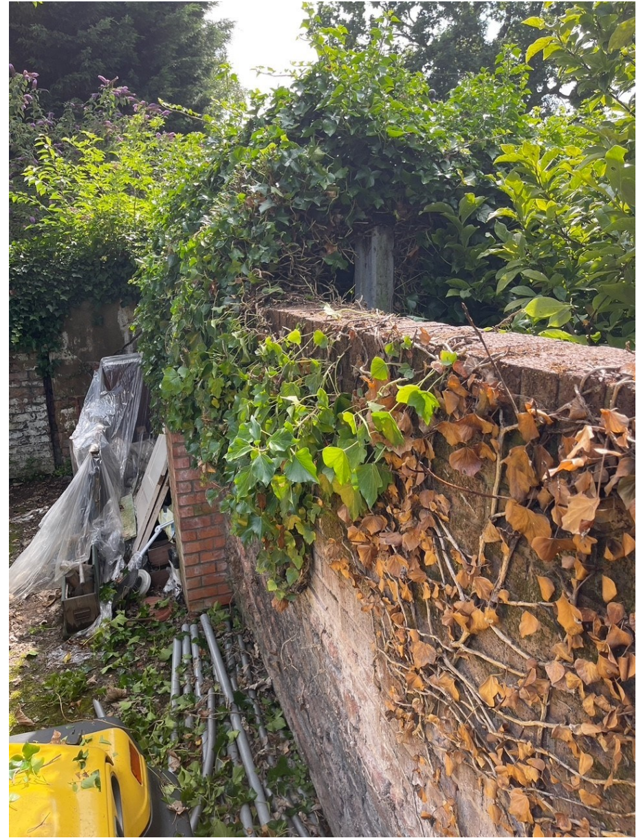
View of wall looking north (no step in the alignment of the wall)
