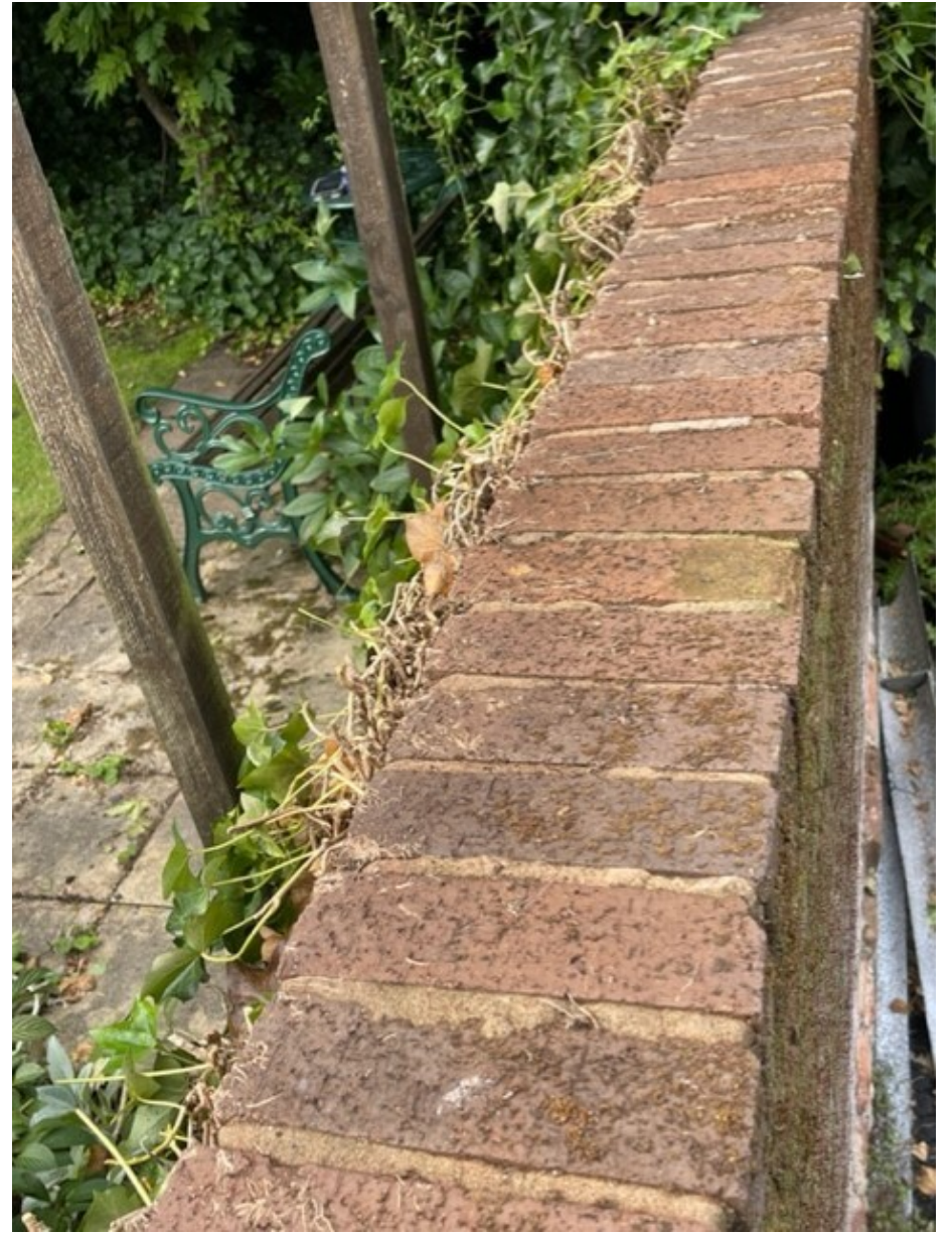
Aerial view of wall looking north (no step in the alignment of the wall)
