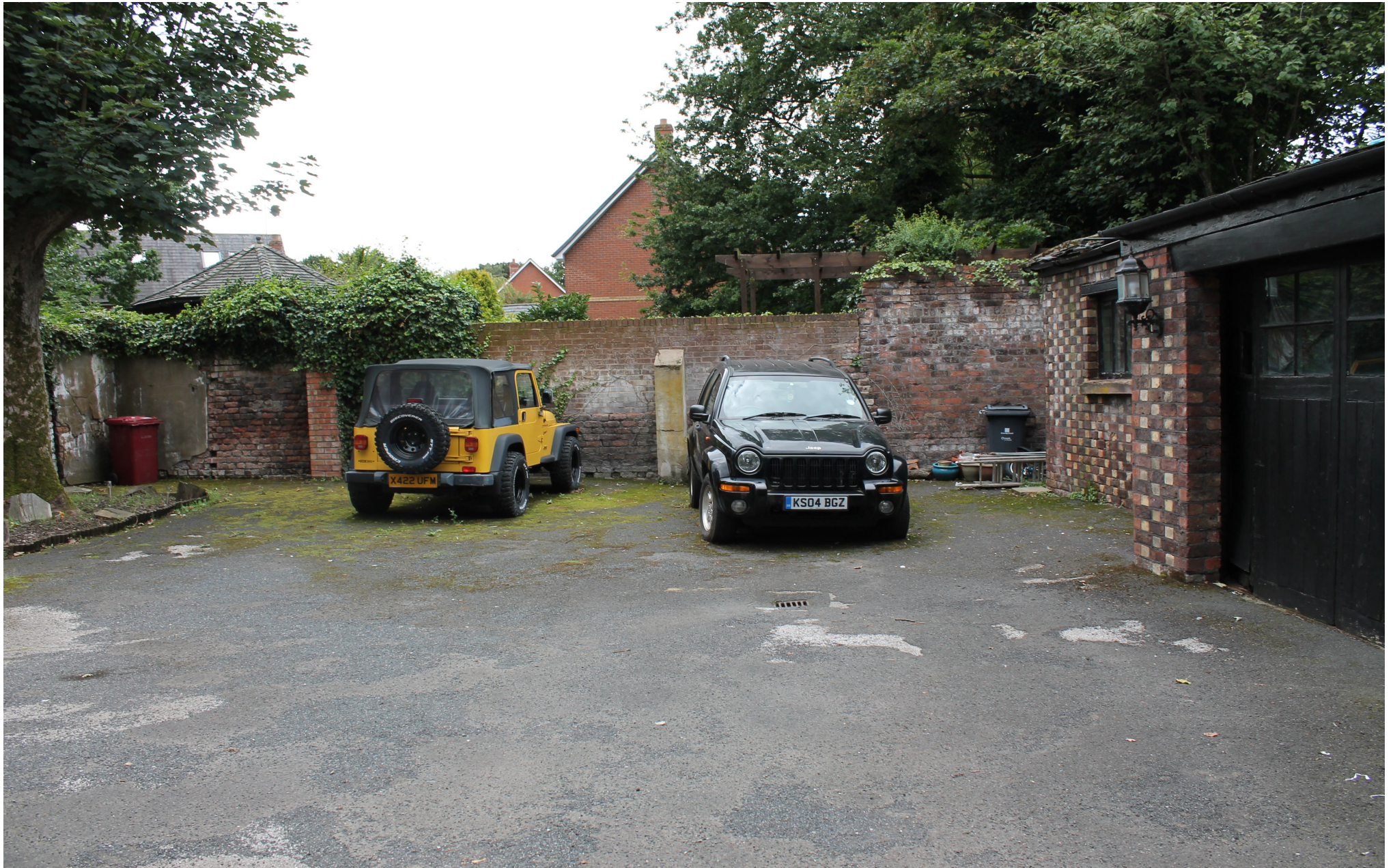
Front facing view of the boundary wall (no step in the alignment at the buttresses)
