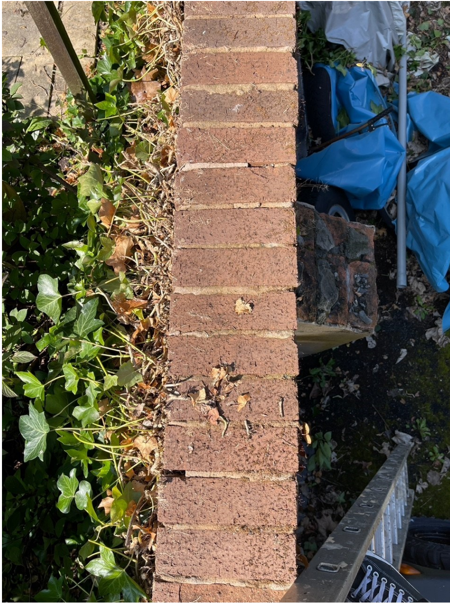
Aerial view of northern buttress (no step in the alignment of the wall)
