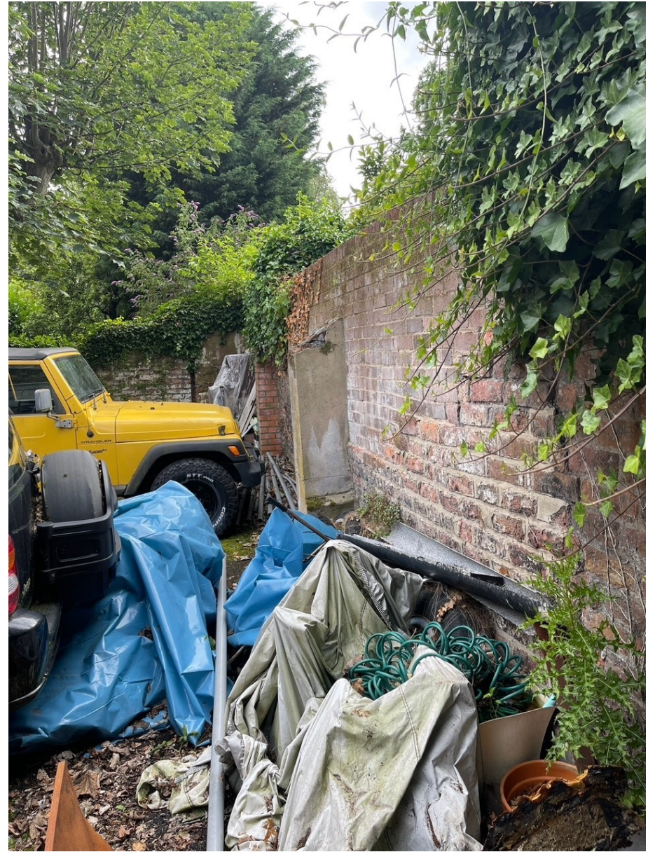
Boundary wall view looking south (no step in the wall at the location of the two buttresses)
