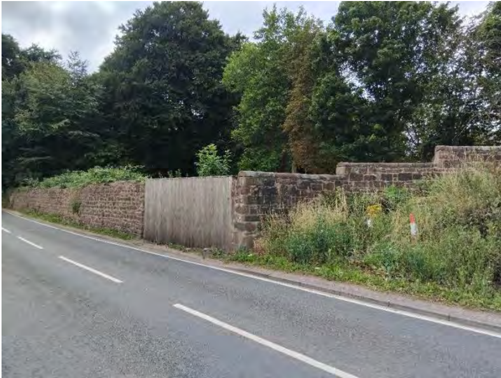
Plate 7. Part of the extant section of former boundary wall which runs along the eastern edge of the study site
