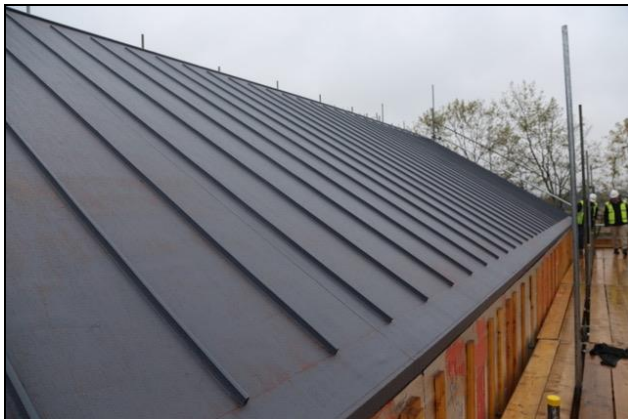
Fig. 1: image of IKO Armourplan PSG single-ply membrane in Slate Grey (RAL: 7015) colour. (Used on a standing-seam pitched roof). Image Source ⇒ Specification Online .
