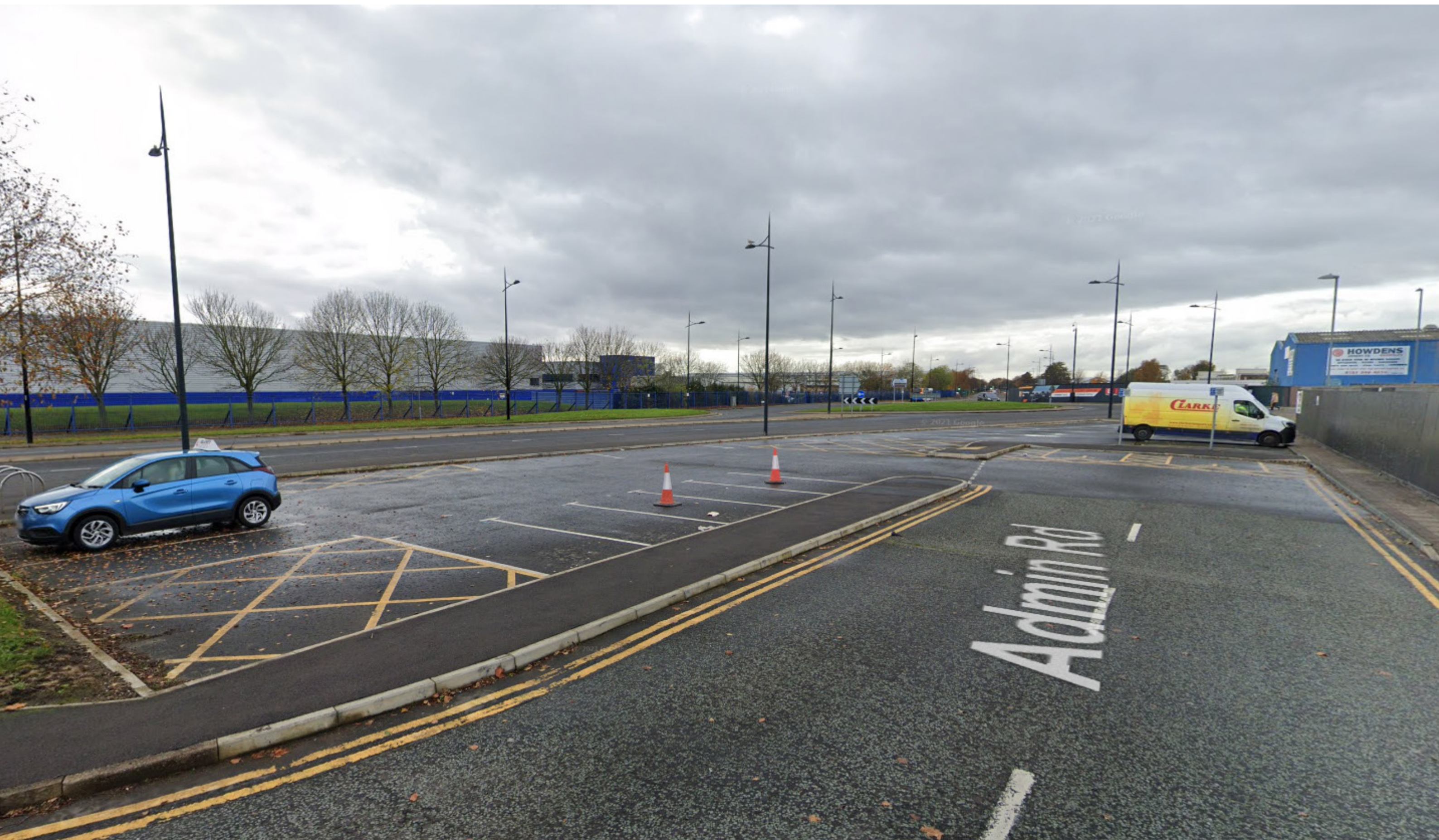
View of existing car park from Admin Road
