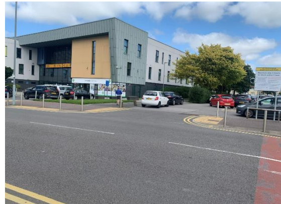
Photograph 2: Existing Site Access
