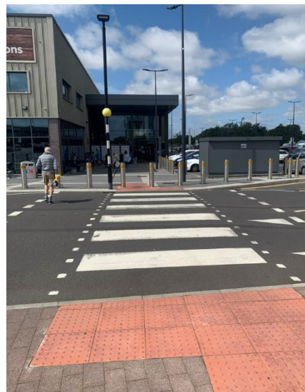
Photograph 15: Irlam Drive Zebra Crossing
