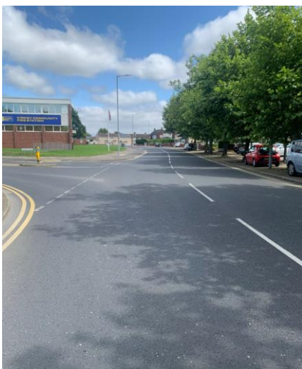
Photograph 5: Webster-Drive Existing Conditions
