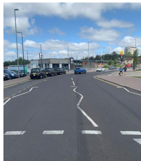
Photograph 6: Irlam Drive Existing Conditions
