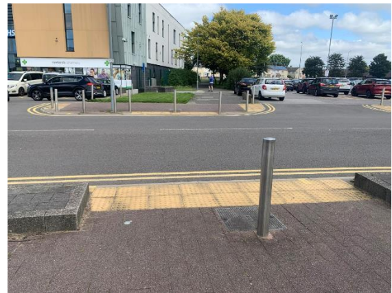
Photograph 12: St Chad's Drive Tactile Crossing
