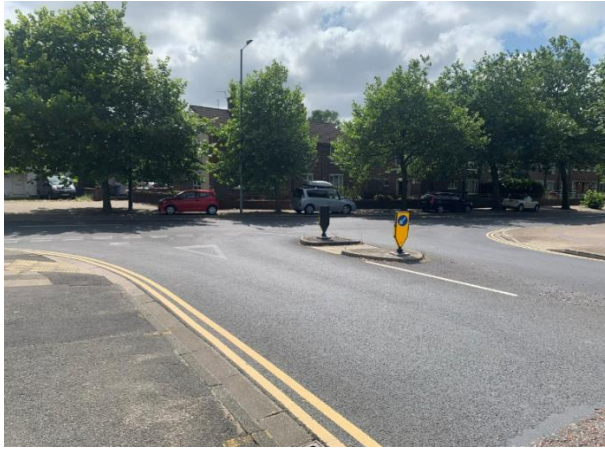
Photograph 13: St Chad's Drive/Webster-Drive Refuge Crossing
