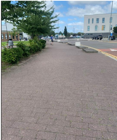
Photograph 7: St Chad's Drive Footway
