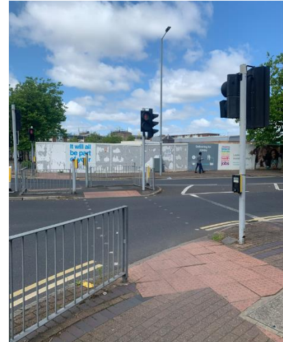
Photograph 14: Webster-Drive/Cherryfield Drive Signalised Crossing
