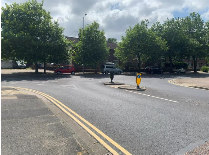
Photograph 13: St Chad's Drive/Webster-Drive Refuge Crossing
