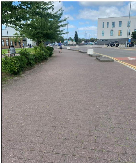
Photograph 7: St Chad's Drive Footway
