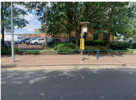
Photograph 16: Eastbound Bus Stop
