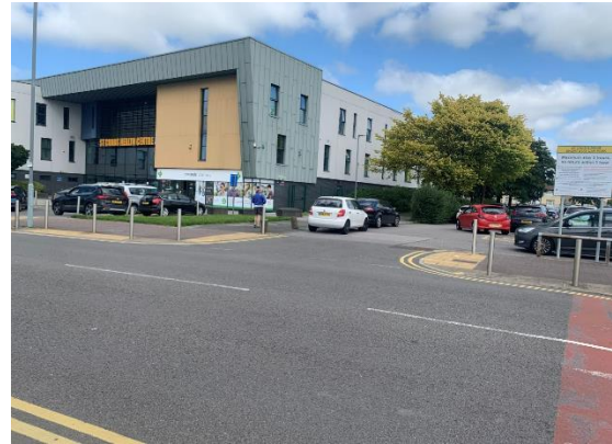
Photograph 2: Existing Site Access
