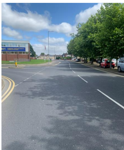
Photograph 5: Webster-Drive Existing Conditions
