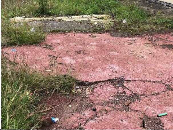
P3: Concrete hardstanding made ground to the west of the site
