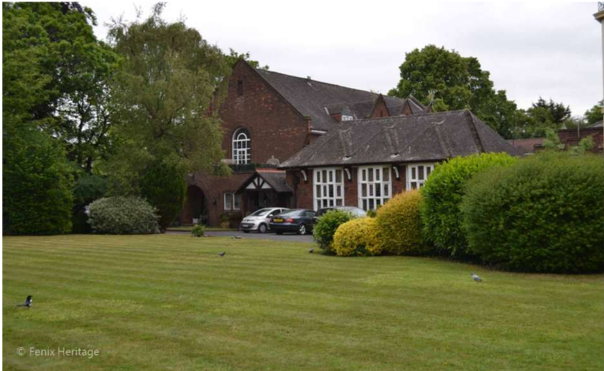
Plate 29: Sightline to the north-east across the lawn to the west of the former Auditorium (a Positive Unlisted Building).
