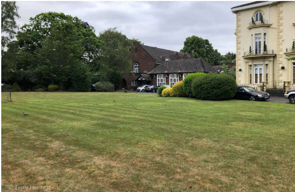
Plate 25: Sightline to the north-east across the lawn to the west of the former Huyton Hall (a Positive Unlisted Building) on the right, and the former Auditorium on the left (a Positive United Building).
