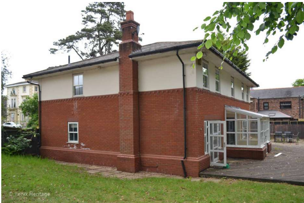
Plate 44: Sightline to the north-east highlighting the existing west-facing and south-facing elevations of the Building.
