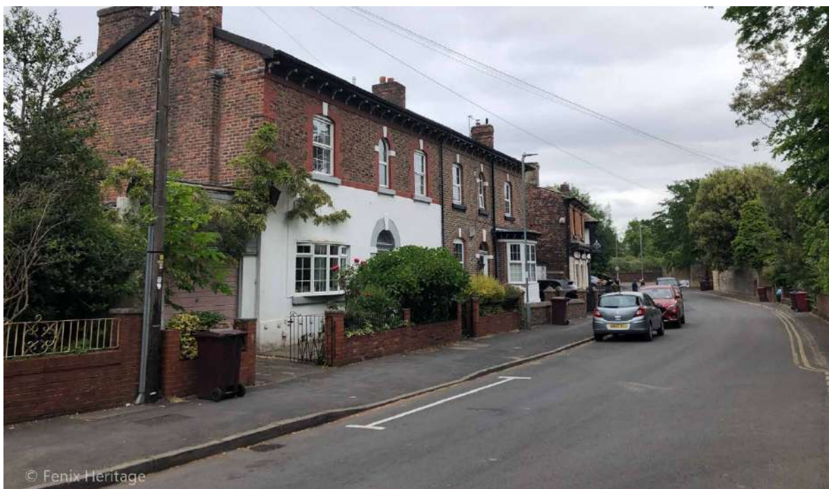
Plate 1: Sightline to the north-east along Blacklow Brow towards The Orchard Conservation Area and the entrance to the former Huyton College complex – now developed as Huyton Hall Crescent. The terraced dwelling to the left is a Positive Unlisted Building with the Conservation Area. The Building is not visible and the proposed development would have no impact on this sightline.
