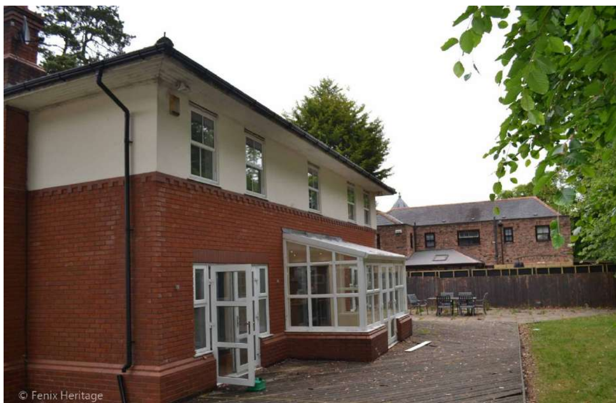
Plate 45: Sightline to the north-east highlining the existing west-facing and south-facing elevations of the Building.
