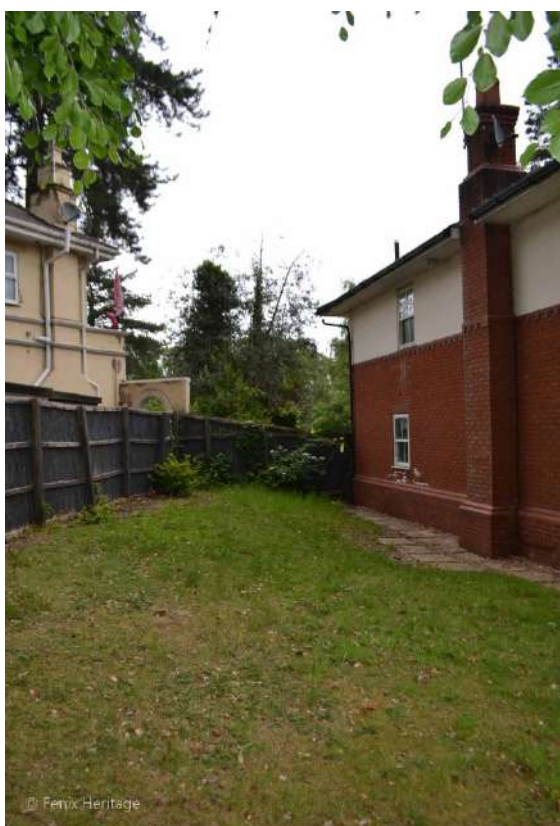
Plate 42: Sightline to the north along the west-facing elevation of the Building. This is the location of the proposed external covered car port and patio.
