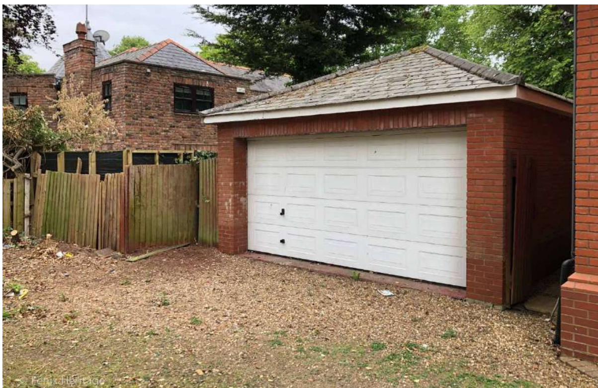
Plate 41: Sightline to the south-west towards the north-facing elevation of the garage.
