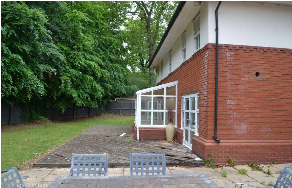
Plate 47: Sightline to the west along the south-facing elevation of the Building. The proposed flat-roofed single-storey extensions for the dining room, kitchen and garden room would occupy this location after removal of the existing conservatory.
