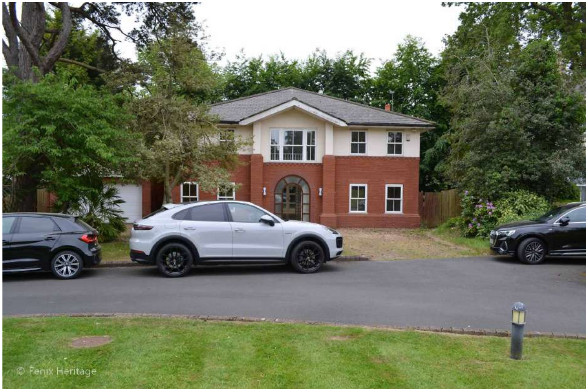
Plate 37: Sightline to the south towards the north-facing elevation of the Building.
