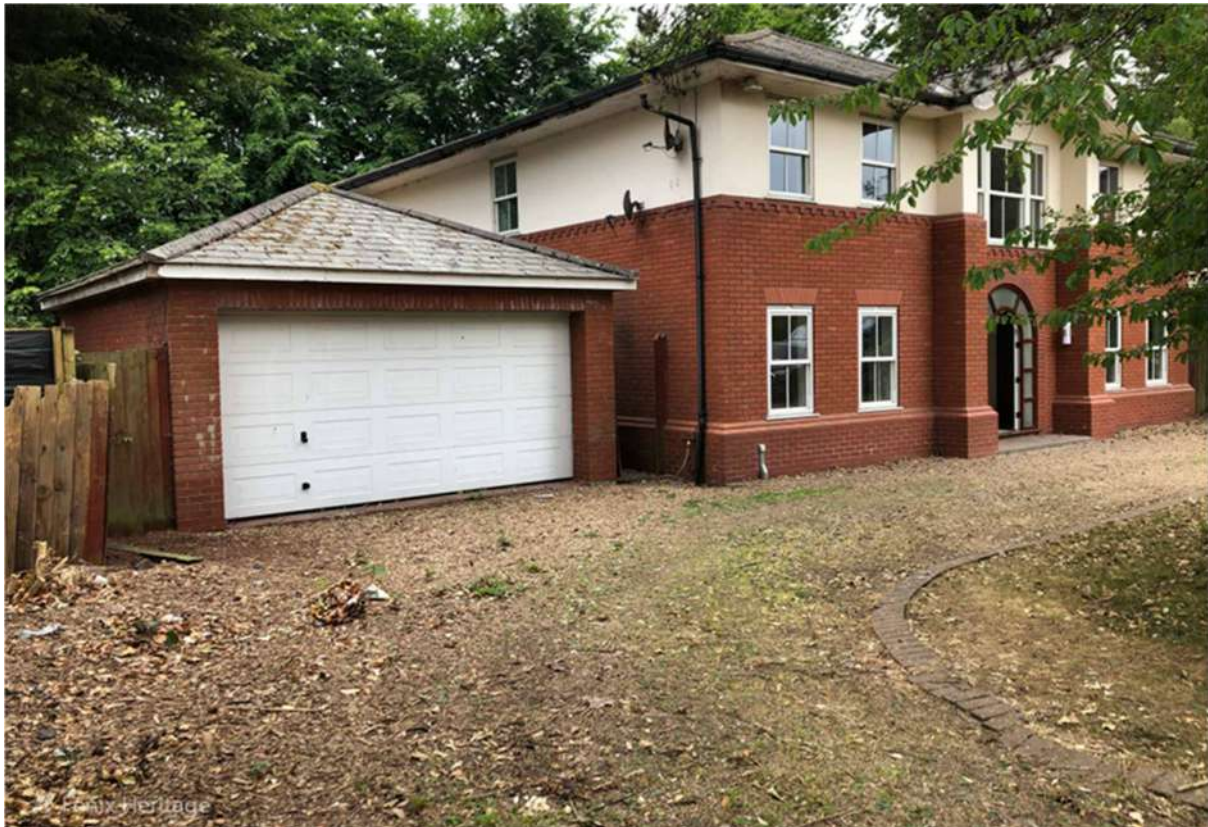
Plate 39: Sightline to the south-west towards the garage and north-facing elevation of the Building.
