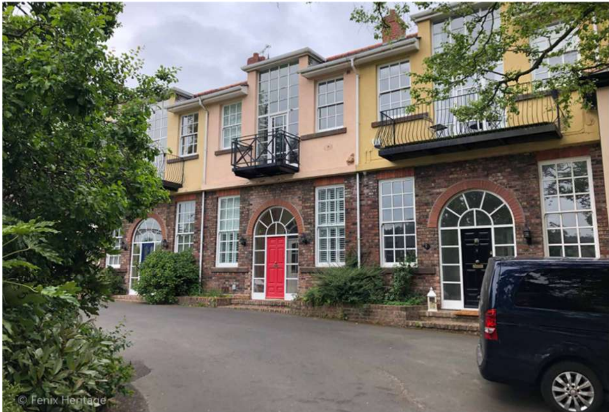
Plate 35: Sightline to the north-east towards the former classroom block of Huyton College. The studio windows are reminiscent of the Listed Building 135-149 Talgarth Road, London, which were built in 1891 as artists' studios.
