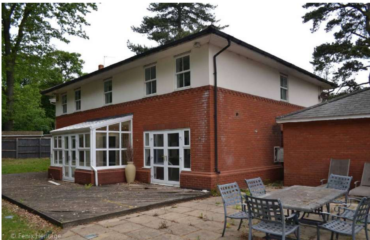
Plate 48: Sightline to the north-west highlighting the existing east-facing and south-facing elevations of the Building and the south-facing elevation of the existing garage.
